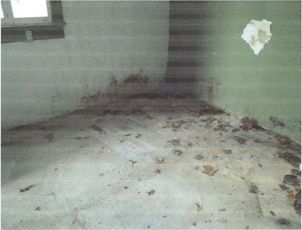
P9 / WATER INFILTRATION AT THE GROUND LEVEL FLOOR
