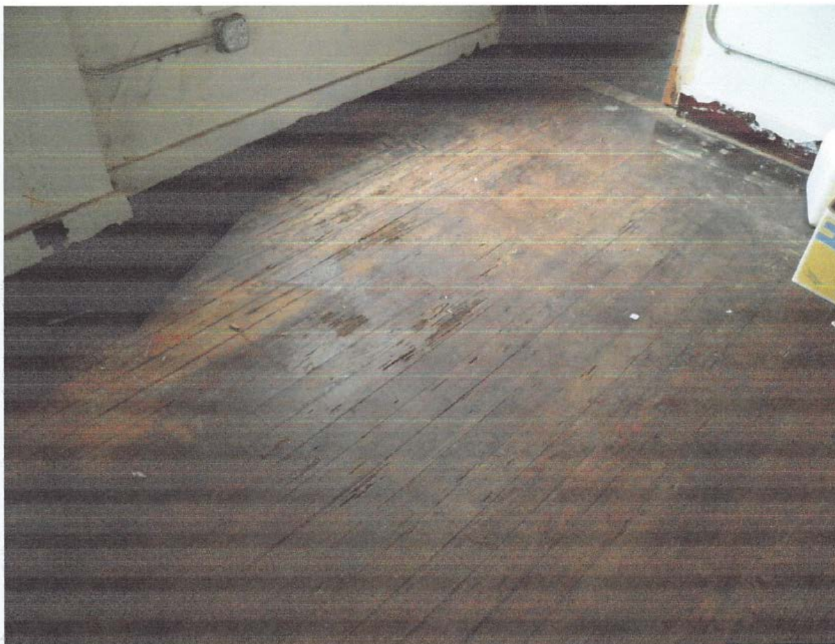
P8 / EVIDENCE OF TERMITE INFESTATION IN THE INTERIOR WOOD
