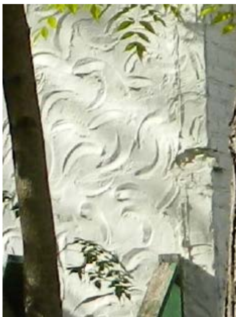
Details of the palm-plastered exterior of the house
