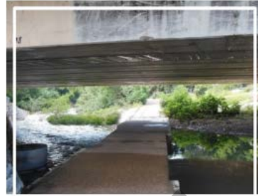
Missing Handrails
