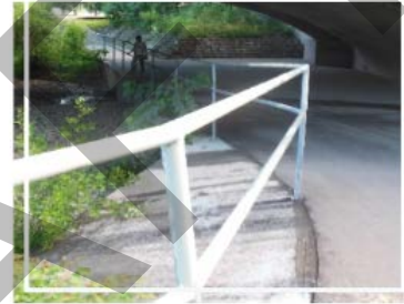
Large Gaps in Handrails
