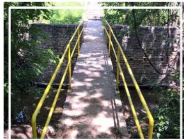
Large Gaps in Handrails
