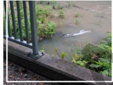
Incomplete Handrails
