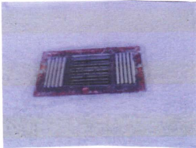
Mold Affected Ductwork
