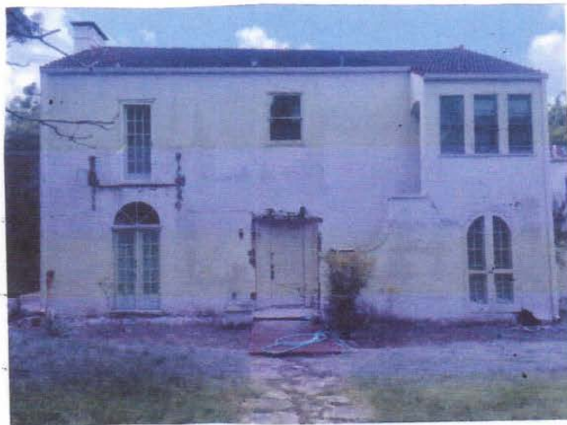
Damaged Exterior Stucco
