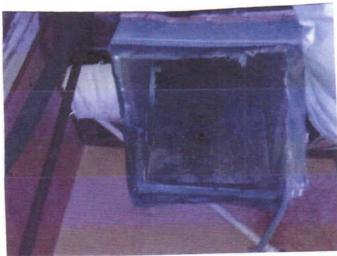
Mold Affected Ductwork
