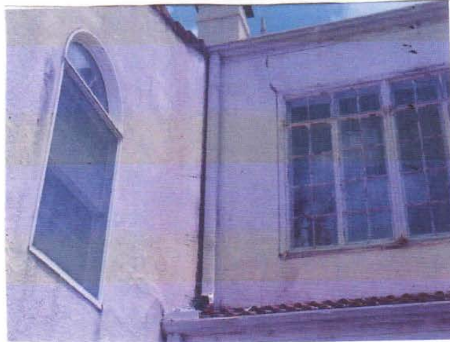
Damaged Exterior Stucco
