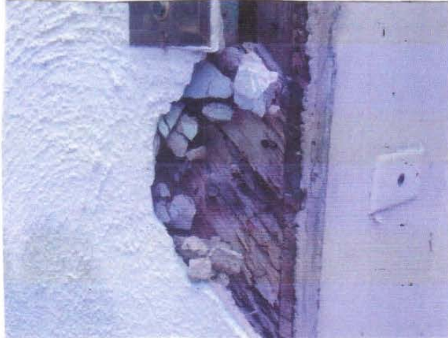
Damaged Exterior Stucco
