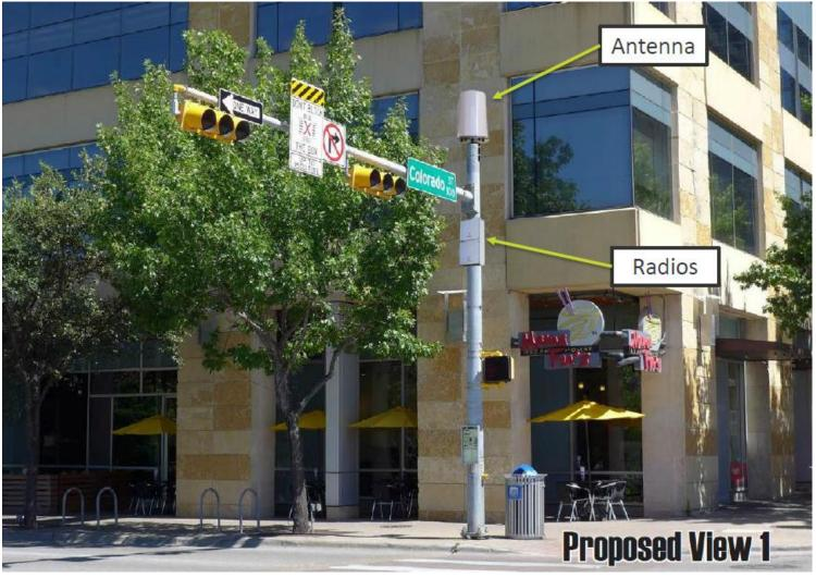
Integrated Antenna & Un-shrouded Radio Module
