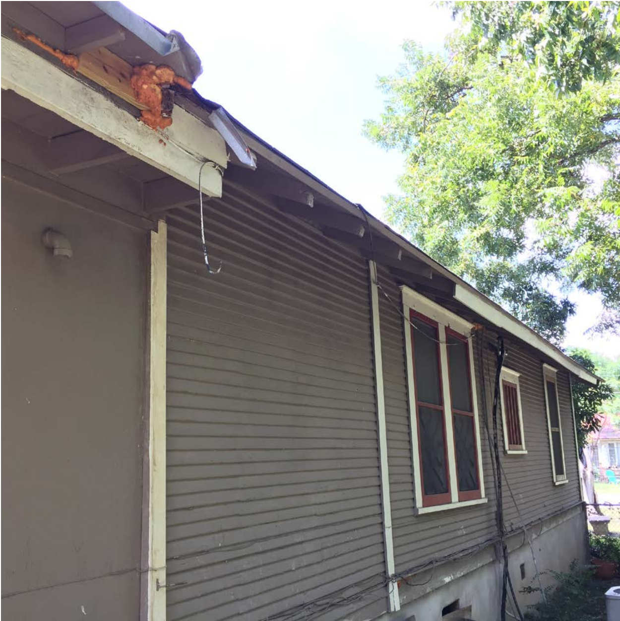
Photos of the house submitted by the applicant for demolition
