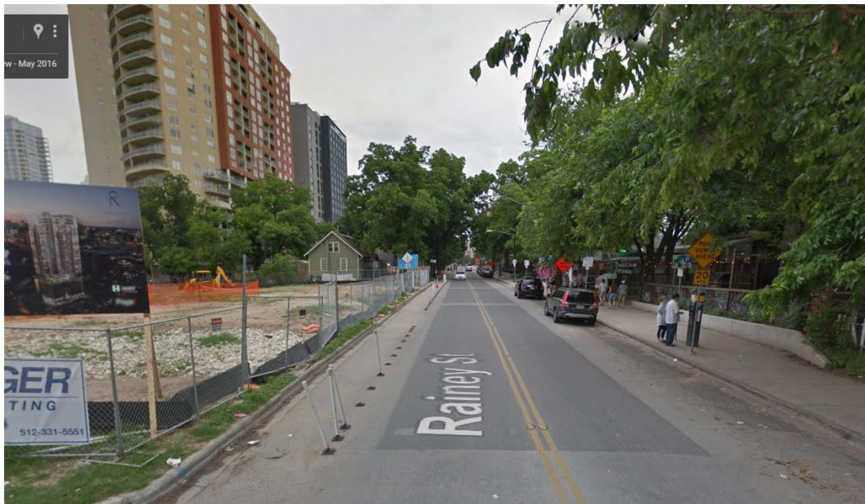
View from the south showing the proposed site on the left. Several of the popular bars and restaurants that have adaptively re-used historic houses are on the right-hand side of the street.
