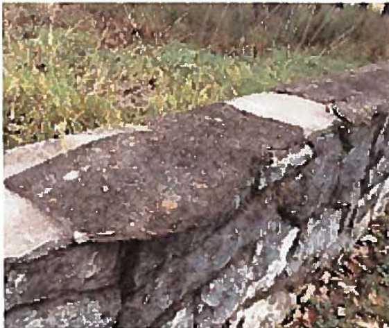
Deteriorated mortar cap
