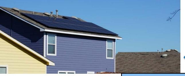
Bunched vents permit solar installation
