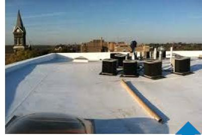
Mechanical equipment and vent clustering to free up roof space
