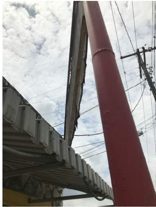
Exhibit 20: Sign not properly supported; falling/flying debris hazard.
