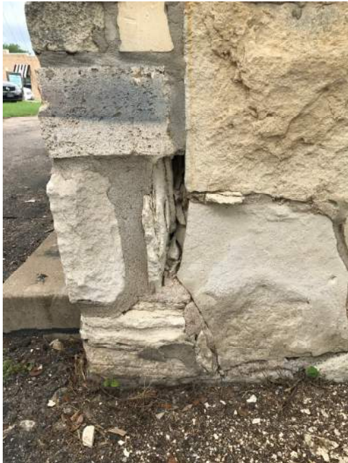
Exhibit 9: Cracking at mortar joints in the rock façade
