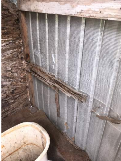
Exhibit 3: Rotting structural members
