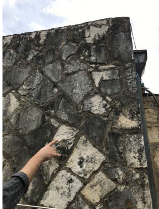
Exhibit 10: Cracking and holes in the rock façade
