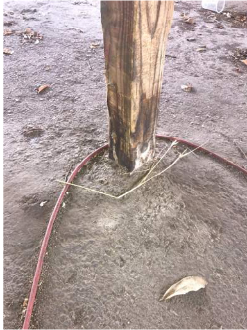
Exhibit 1: Improper column connection
