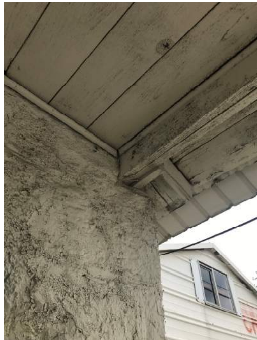
Exhibit 16: Inadequate bearing condition
