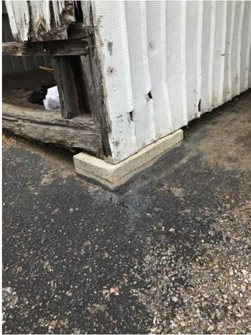
Exhibit 7: Improper foundation
