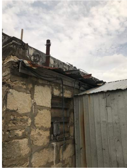
Exhibit 18: Metal roof deck warping
