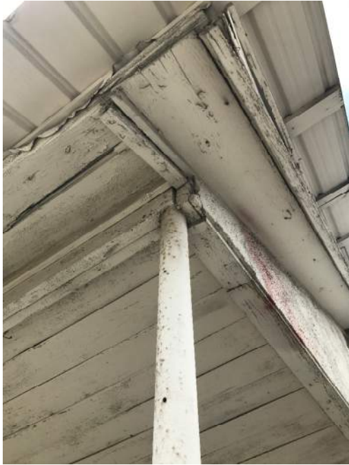
Exhibit 5: Inadequate connection at top of column
