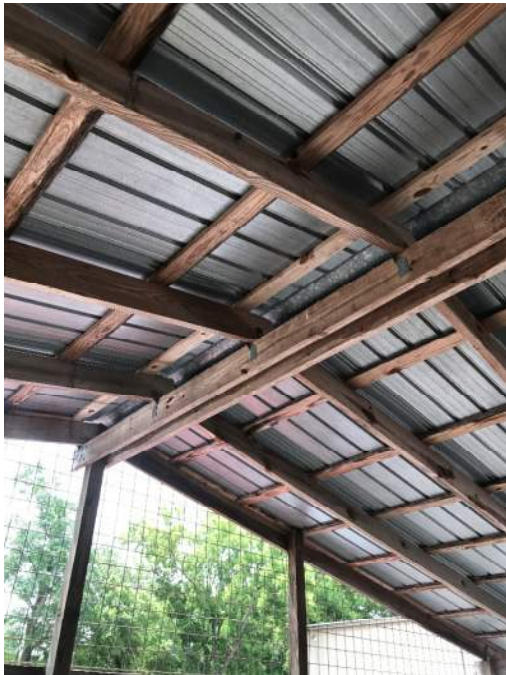
Exhibit 2: Improper rafter connection for transfer of lateral loads and stability
