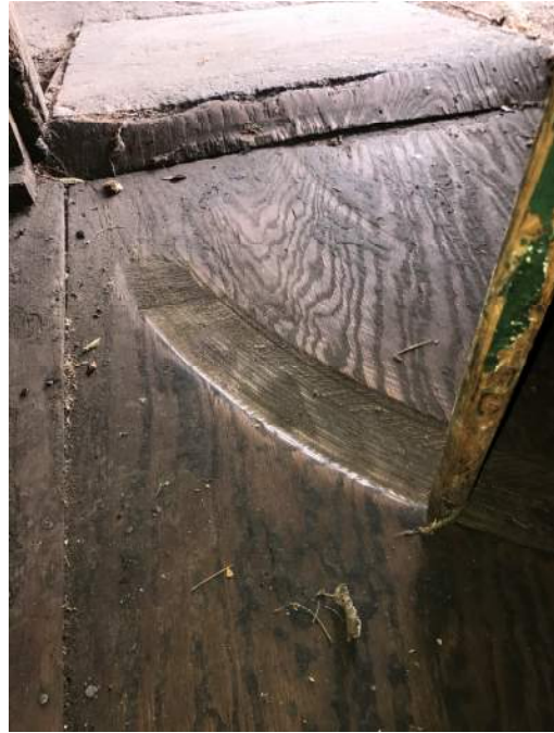
Exhibit 14: Floor settlement and uneven floors
