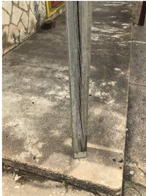
Exhibit 13: Significant checking of wood post
