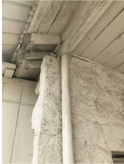
Exhibit 5: Inadequate connection at top of column
