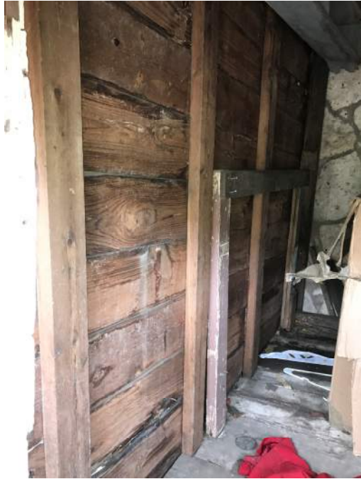
Exhibit 17: Improper stud wall framing
