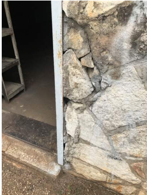
Exhibit 9: Cracking at mortar joints in the rock façade
