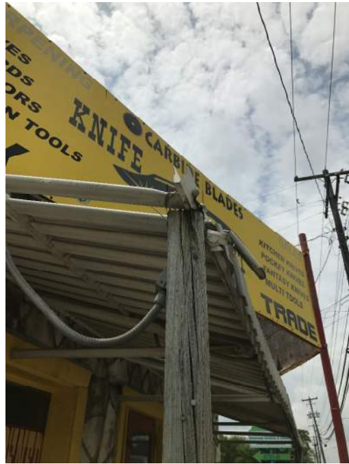
Exhibit 12: Column connection to canopy inadequate
