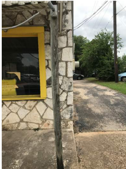
Exhibit 19: Wood column warping, deteriorating at base.
