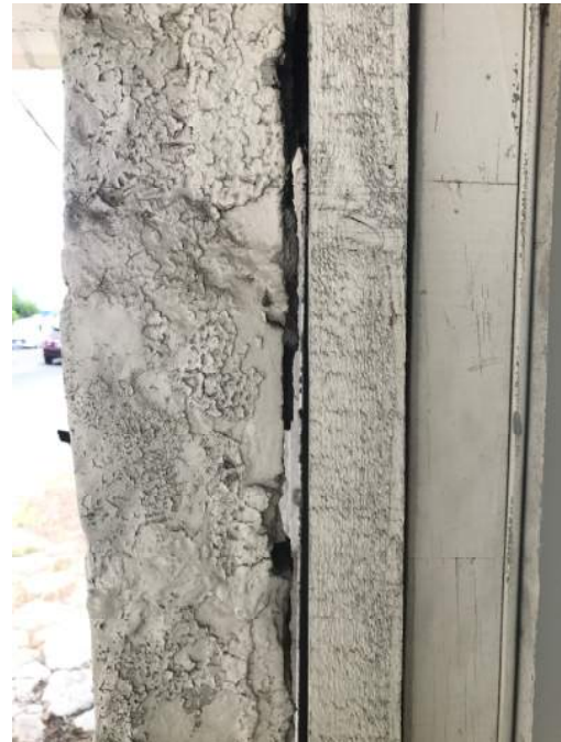
Exhibit 6: Stone façade potentially unsupported by wall
