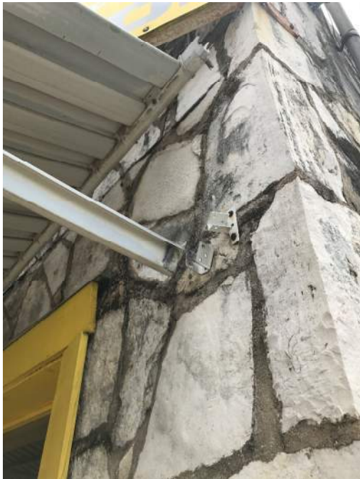
Exhibit 11: Canopy connection failures
