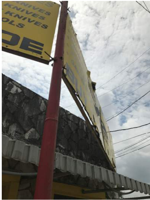
Exhibit 20: Sign not properly supported; falling/flying debris hazard.
