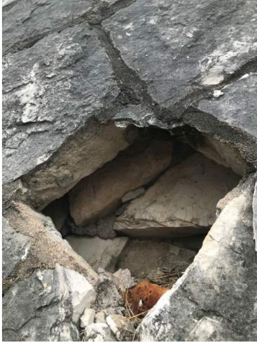
Exhibit 10: Cracking and holes in the rock façade
