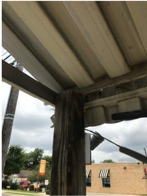
Exhibit 12: Column connection to canopy inadequate
