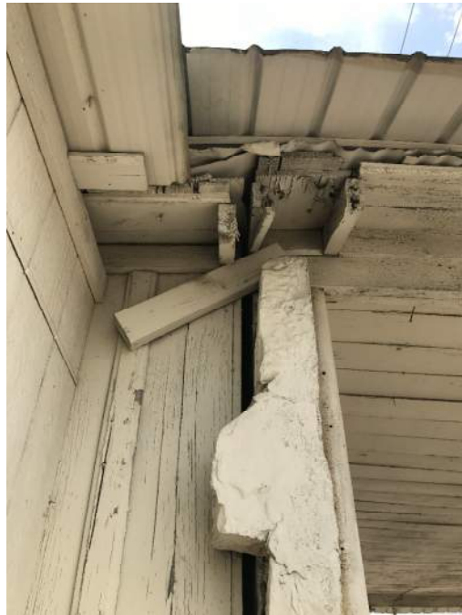
Exhibit 6: Stone façade potentially unsupported by wall
