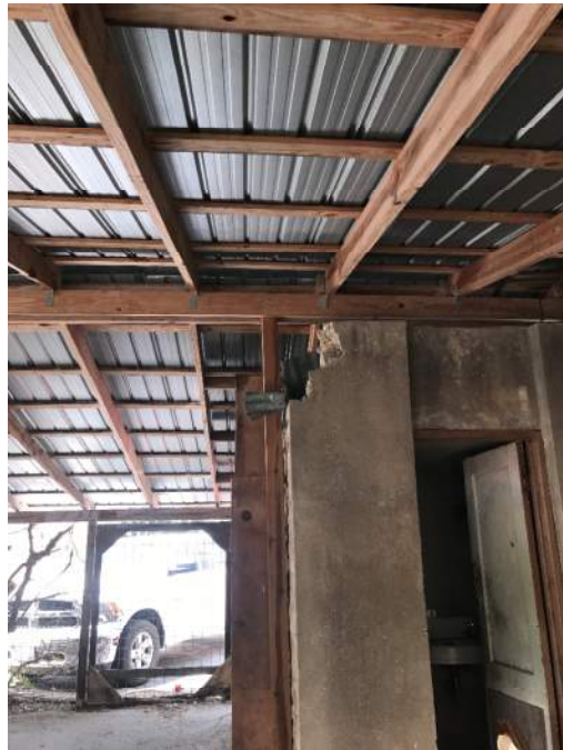
Exhibit 21: Spalled concrete Wall
