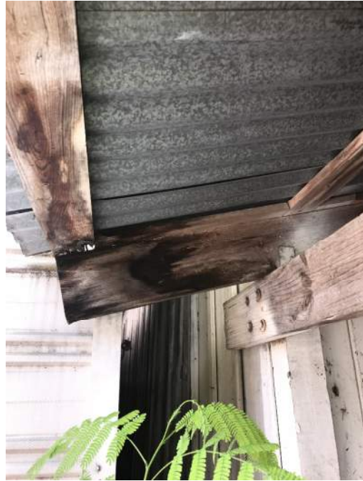
Exhibit 3: Rotting structural members
