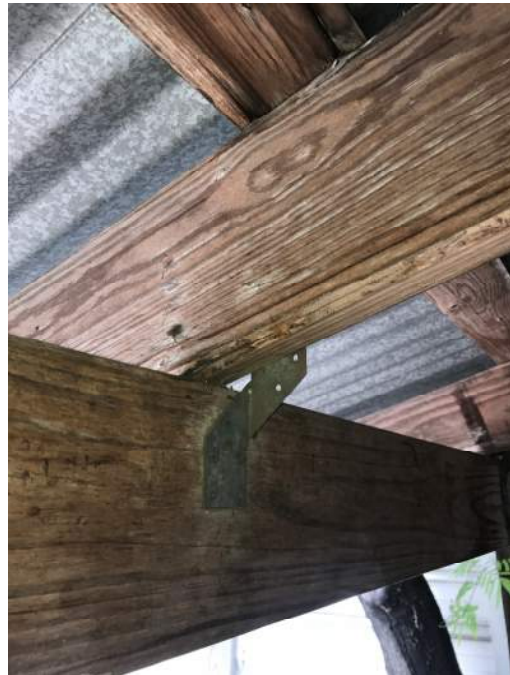
Exhibit 2: Improper rafter connection for transfer of lateral loads and stability
