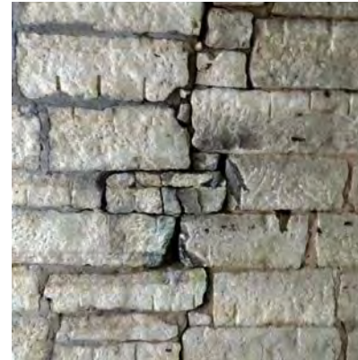
Broken stone / Missing mortar
