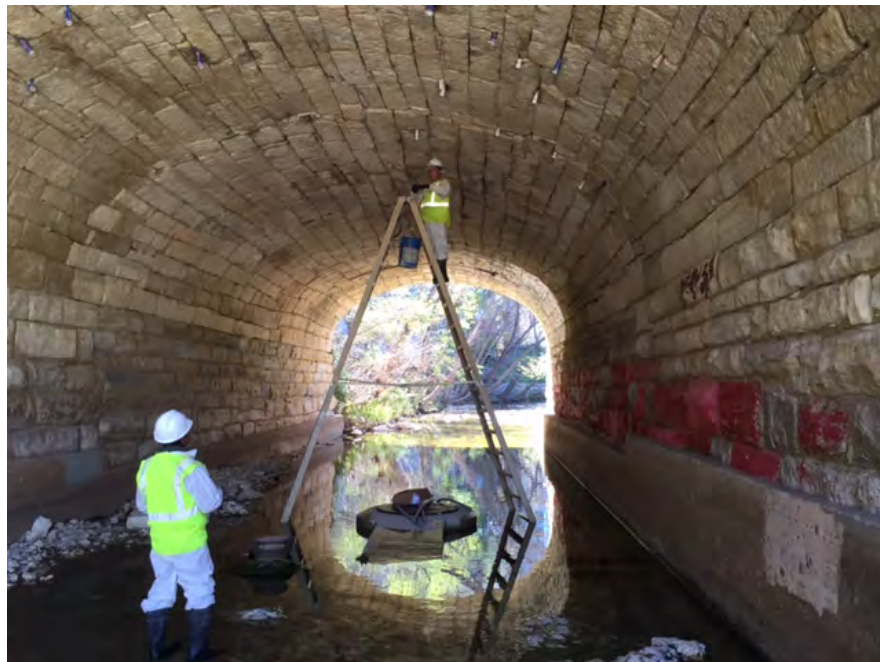
Regrouting of the bridge in 2016. The little tubes inserted in between the stones are escape chutes for the bridge's resident bats.
