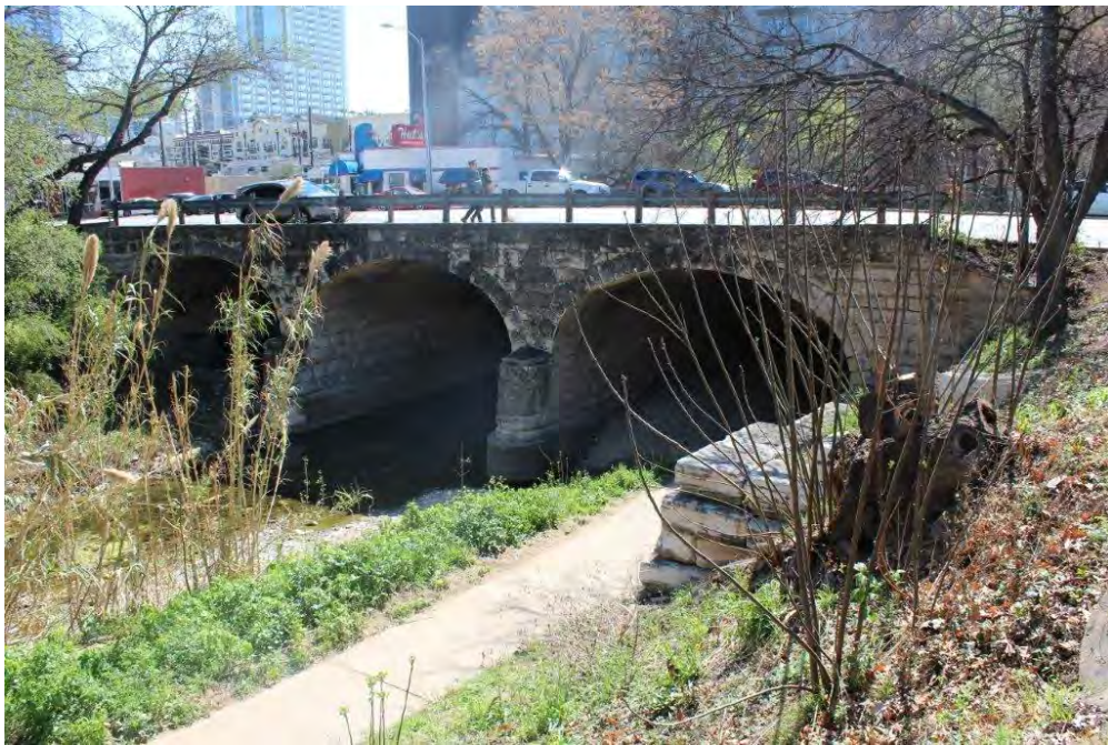
West 6 th Street Bridge, north face. The metal guardrail installed in place of the destroyed parapet is visible here. The northwest retaining wall made of large stone blocks is visible on the right side of the photo.
