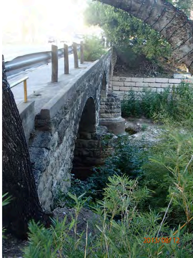
Another view of the bridge's north side and metal guardrail. The northwest retaining wall is visible here on the right side of the photo.
