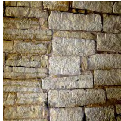
Construction joint - change in stone -
