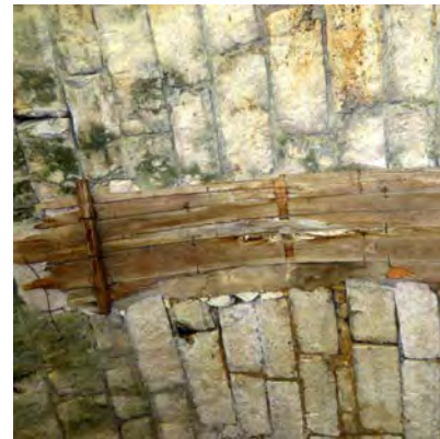
Utilities cut into arch stones
