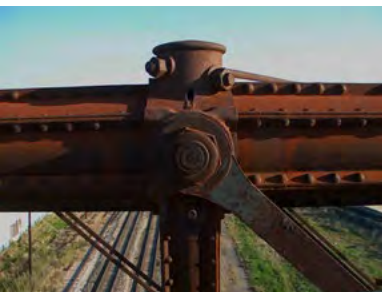
Above: Upper chord pin and eyebar connection, during assessment.
