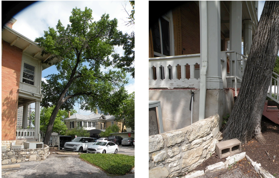
Figure 13 - The cedar elm at the southwest corner of the building is causing structural damage, and must be removed.
