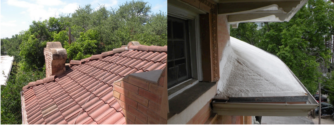
Figure 8 - Existing roof systems over the porte cochère and main house.
