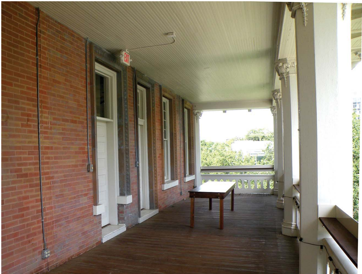
Figure 7 - Exposed conduit will be concealed, floors will be replaced, and additional masonry cleaning and conservation will be performed at the second floor porch
