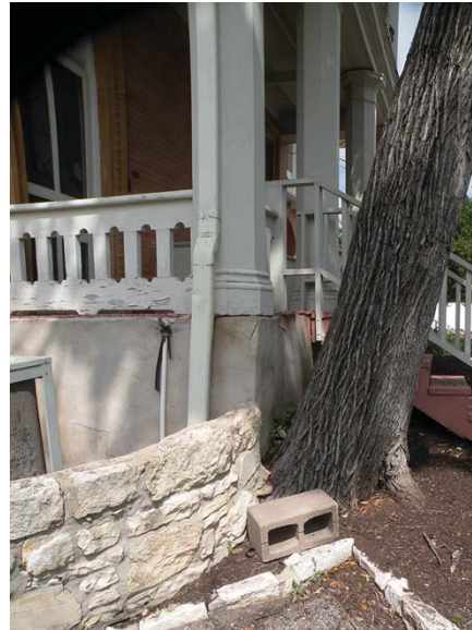
Figure 13 - The cedar elm at the southwest corner of the building is causing structural damage, and must be removed.
