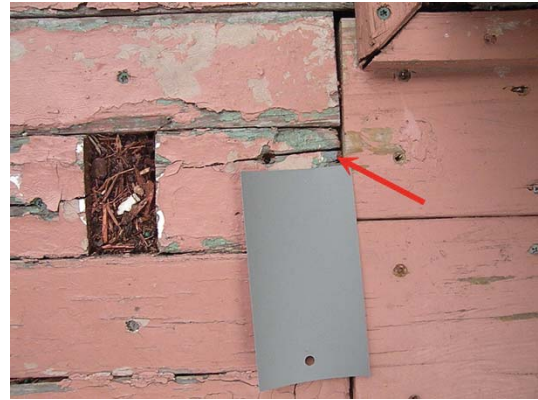
Figure 6 - Deteriorated wood floors will be replaced; paint color will match historic.
