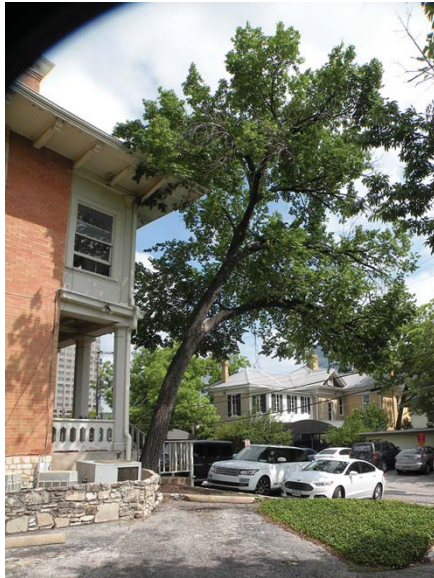
Figure 13 - The cedar elm at the southwest corner of the building is causing structural damage, and must be removed.
