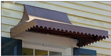
The decorative, flared copper awning over the window provides protection from the elements.
