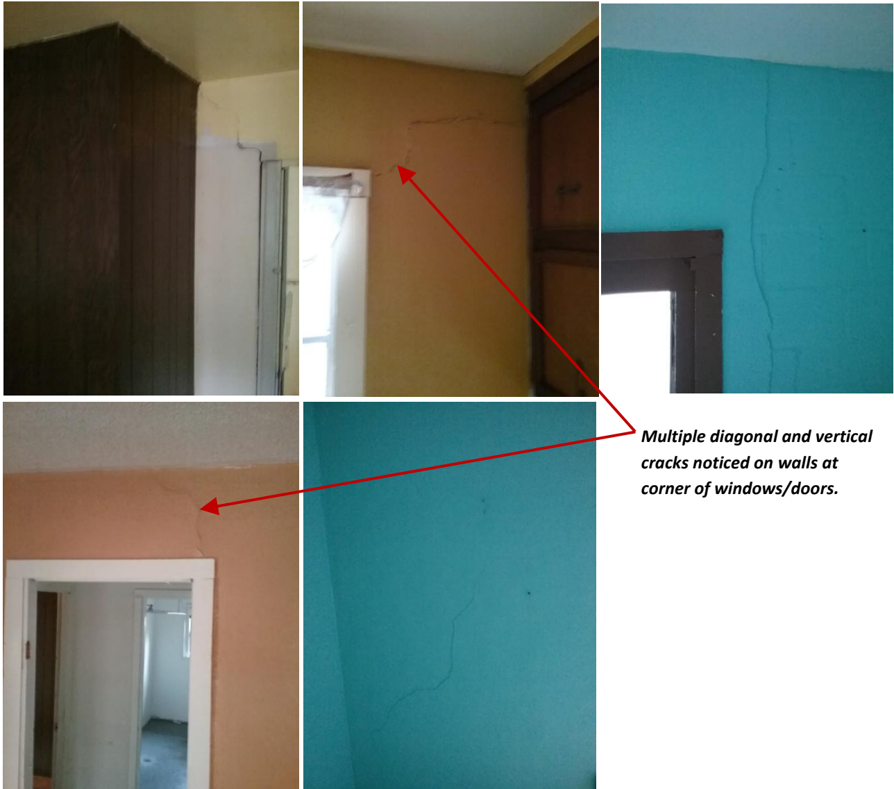
Figure 3: Cracks in walls
