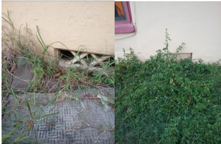
Figure 1: Limited crawl space access
