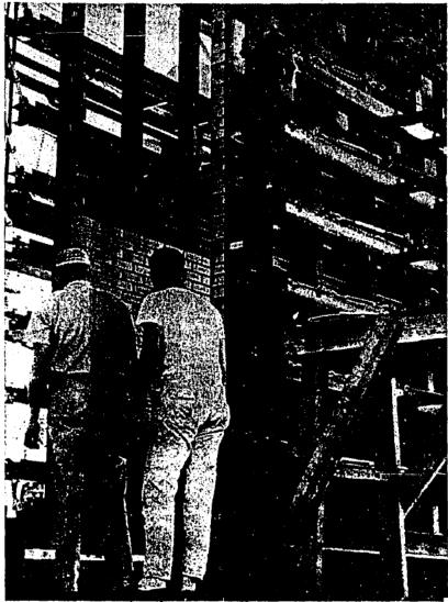
NEW BRICK WALL PROCESS—A vertical brick-laying machine, first of its kind in the world, forms a 12 by 12 foot reinforced wall at the Elgin Standard plant near Elgin. The giant machine, which resembles an oversize waffle iron, can form the bricks or any other masonry material into varying patterns at the rate of 2,000 per hour. Developed by W. W. Coates and
