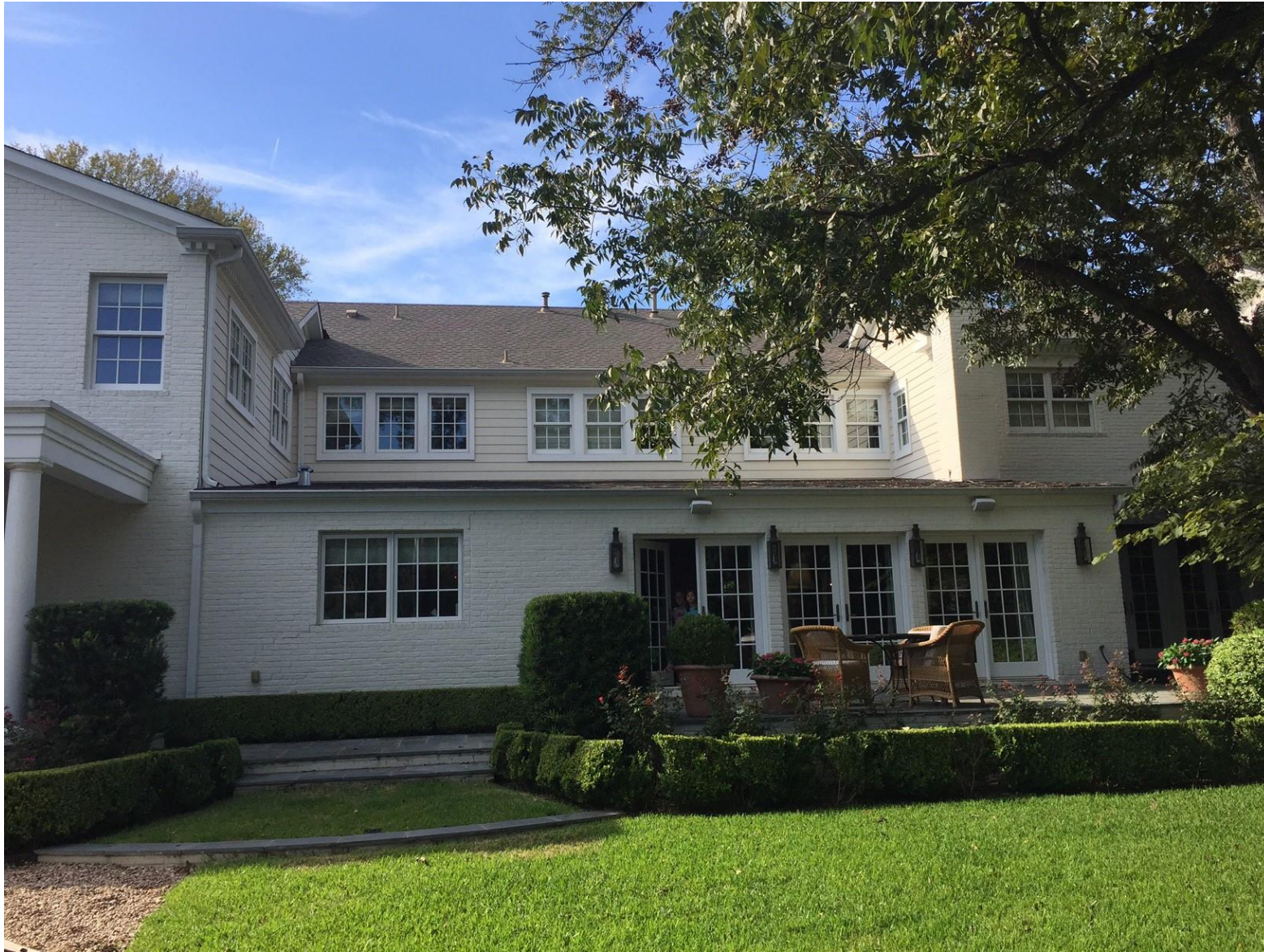
Rear (east) elevation, center view. The second-story inset is proposed to be infilled. The ground floor level under this inset is a previous non-historic addition (ca. 2006-08).
