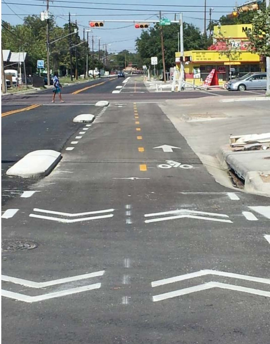
Austin, Texas, Pedernales Street – Cast in Place Barrier Curbs with Breaks for Inlets and Driveways
