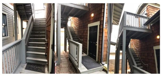
This is the existing stairwell to the second story garage apartment. This stairwell to be torn down, removing significant mass from the structure.
