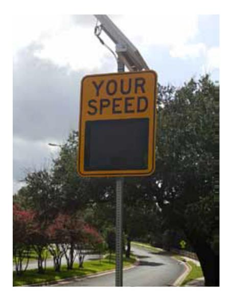
Measures & displays the speed of vehicles, typically paired with a speed limit sign
