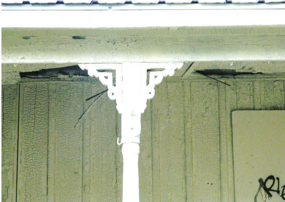
2018 photograph showing porch bracket detail and damage to porch ceiling.
