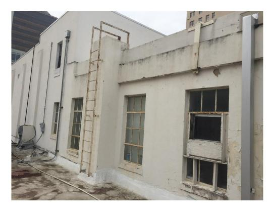
Significant flaking, blistering, and general deterioration of stucco. All problem areas to be fully removed and replaced with an approved and much more durable stucco.
