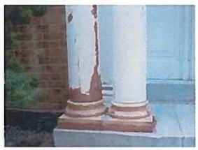
Deteriorated wood parch elements can be repaired in place with epoxy consolidants and fillers.
