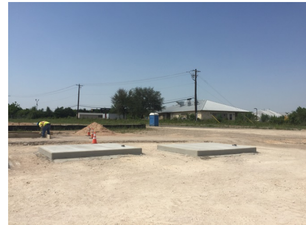
Figure 6: Battery foundations ready
