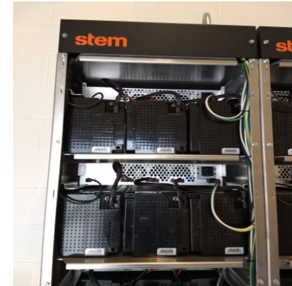
Figure 3: 1kW battery packs
