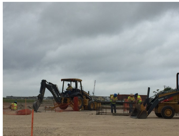
Figure 5: Crews working on rebar structures for battery foundations
