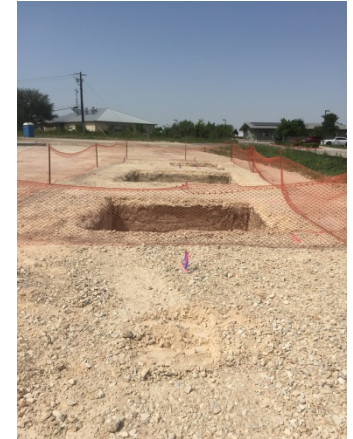
Figure 3: Prep work for interconnection foundations
