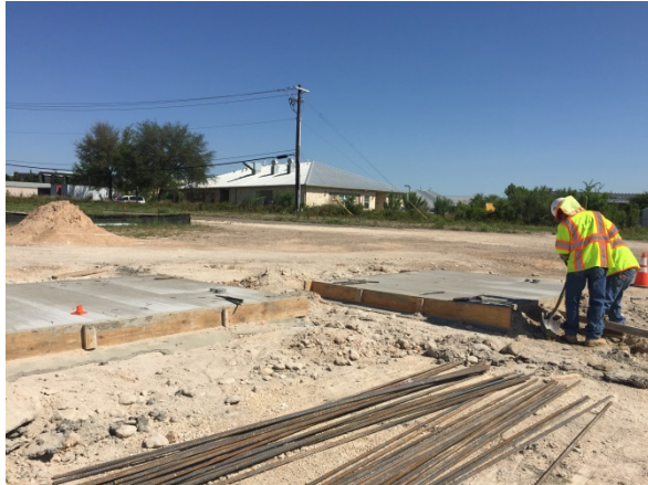
Figure 1: Crews working on rebar structures for battery foundations
