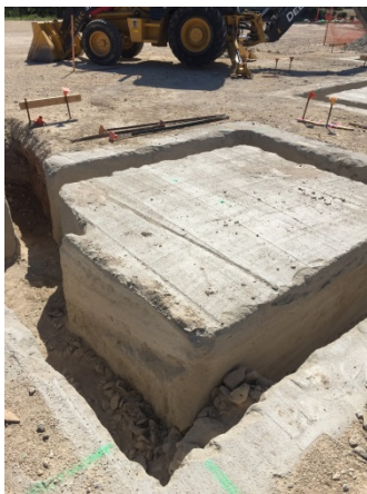
Figure 4: Battery foundation
