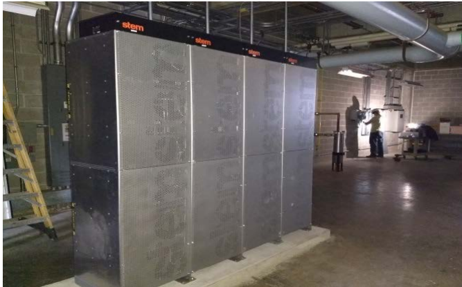
Figure 1: 72kW/144kWh commercial battery
