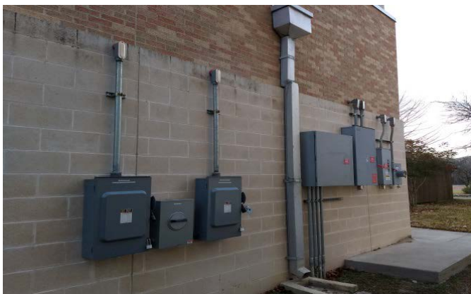
Figure 4: External interconnection equipment for solar and storage
