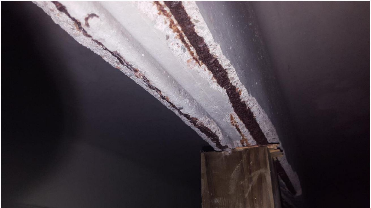
Exposed and corroded rebar with temporary shoring.
