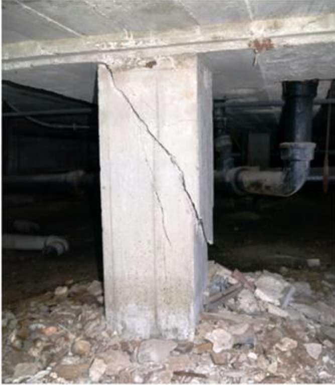
Shear column – damaged
