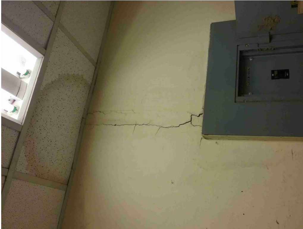
Interior wall and roof – cracking and water damage
