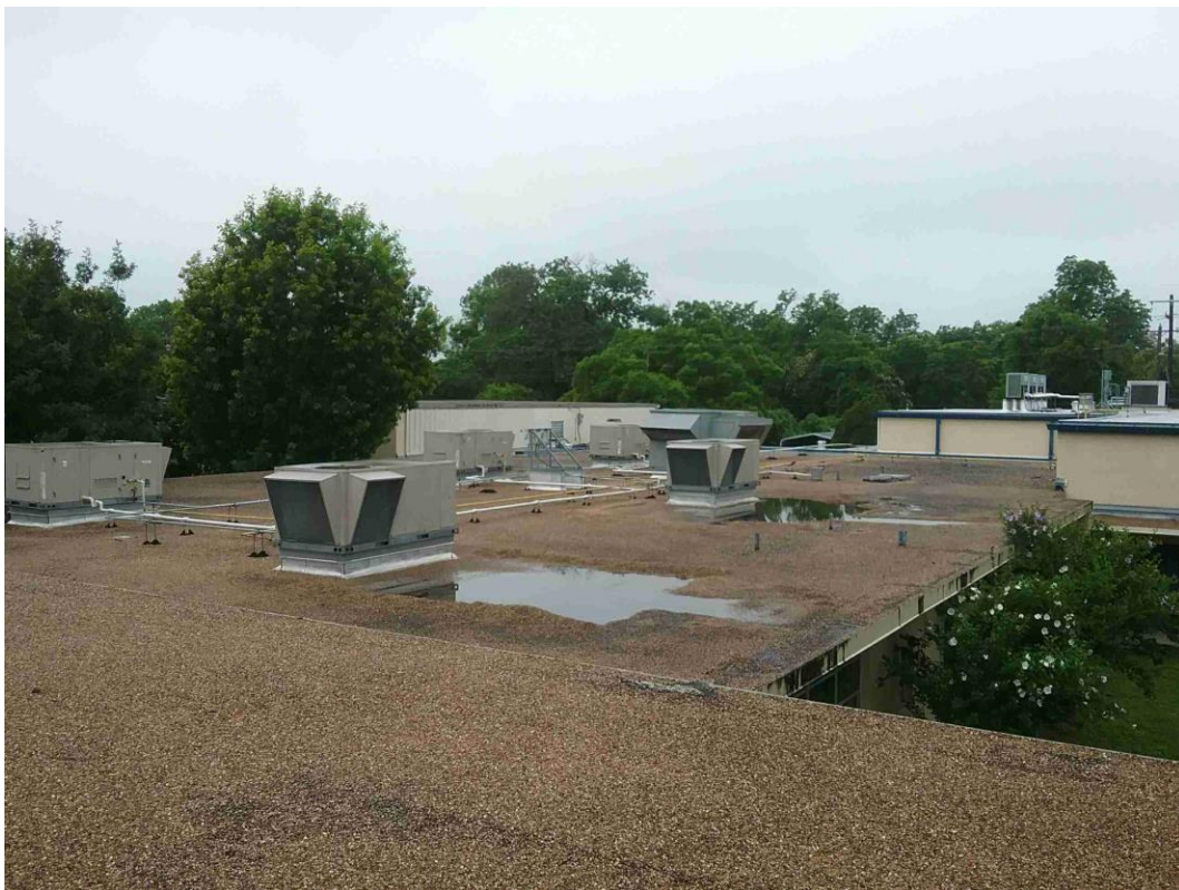
Roof – corrosion and water damage from ponding
