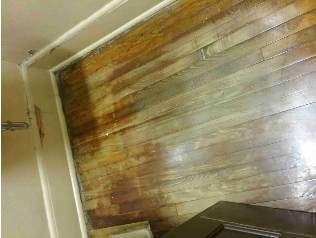
Aged and damaged flooring
