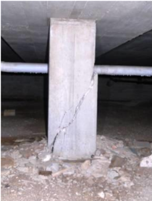
Shear column - damaged
