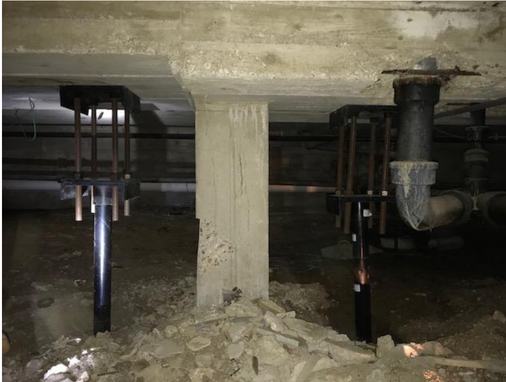
Shoring to temporarily stabilize structure installed.
