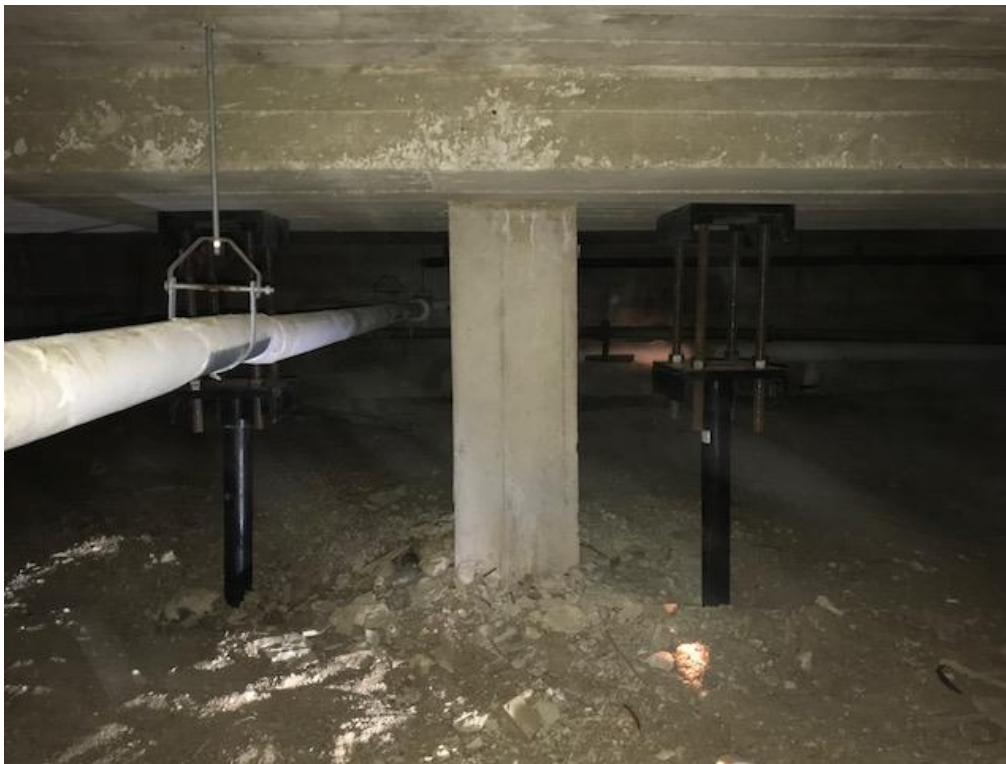
Shoring to temporarily stabilize structure installed.
