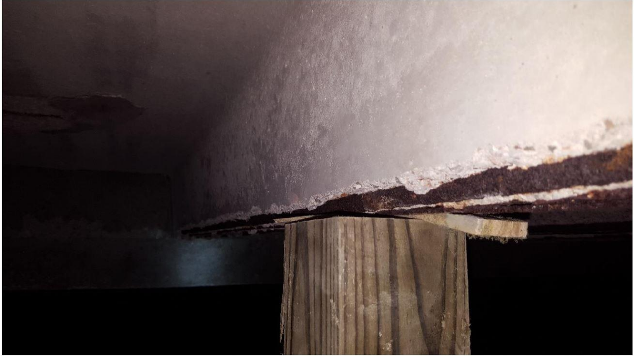
Exposed and corroded rebar with temporary shoring.
