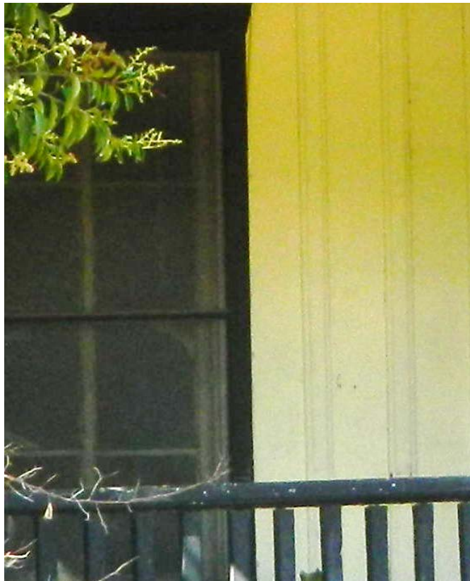
Detail of 4:4 front window and board-and-batten siding on the front porch.
