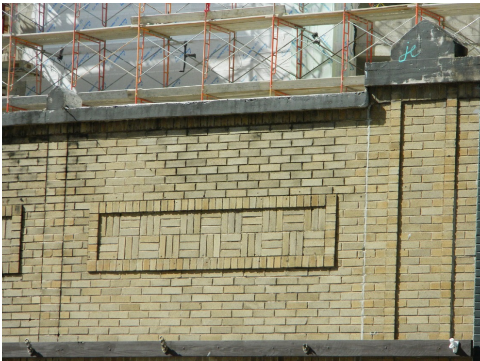
Detail of decorative brickwork in the parapet and cast stone coping and pier cap (July, 2018)
