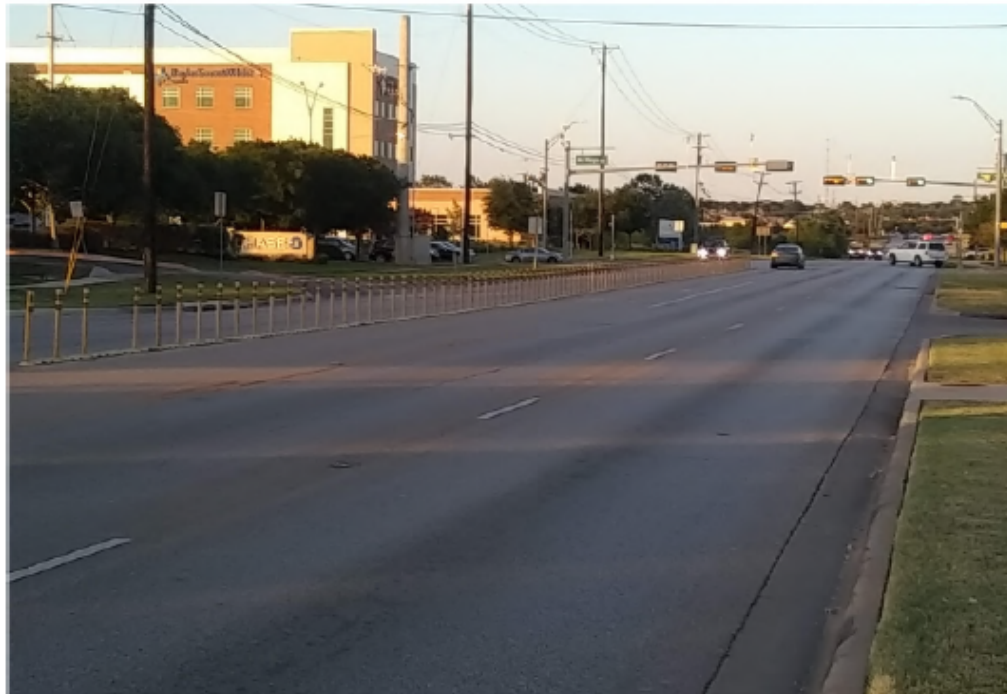
SURFACE MOUNTED DELINEATORS • UNIVERSITY BLVD AT MAYS ST, ROUND ROCK
