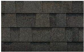
Composition shingle roofing
