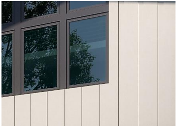
Painted reverse board and batten siding
