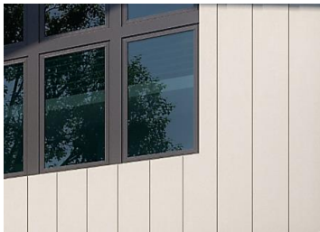
Painted reverse board and batten siding
