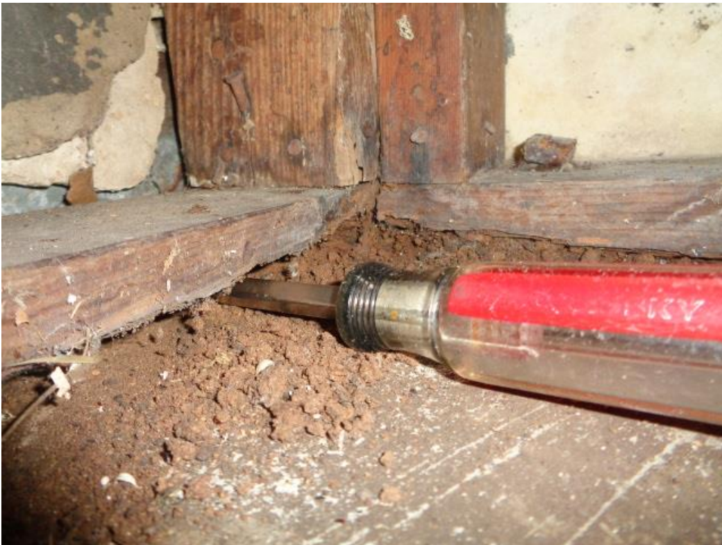
Photo 9: The damage from subterranean termites at the bottom sill in the right rear storage room.
