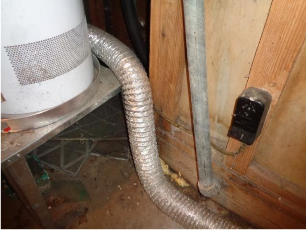
Photo 42: The dryer flue is not rigid metal as required.
