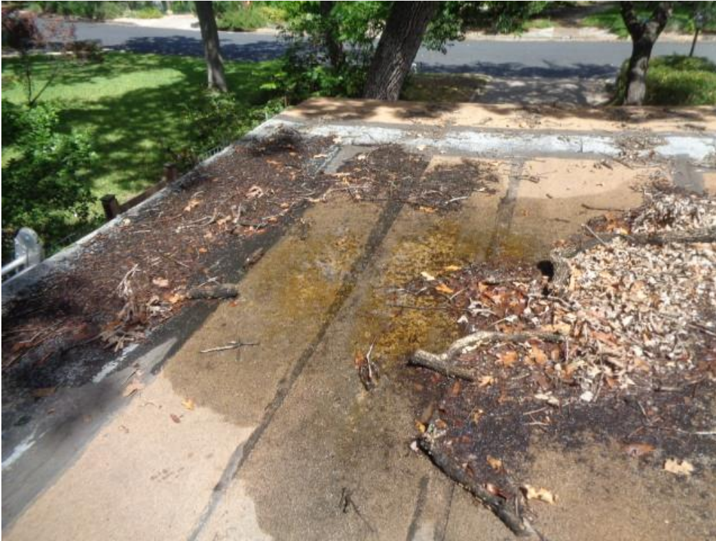
Photo 22: The ponding on the carport roof.
