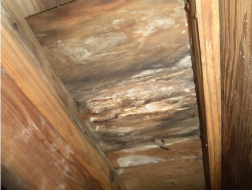
Photo 2: The water damaged subfloor under the front bathroom shower.
