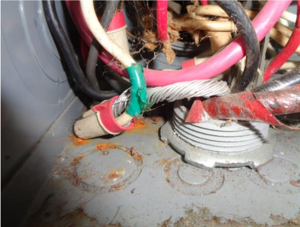
Photo 32: The silver wiring that is spliced in the rear exterior wall subpanel - make sure this is not an aluminum/copper wire splice.
