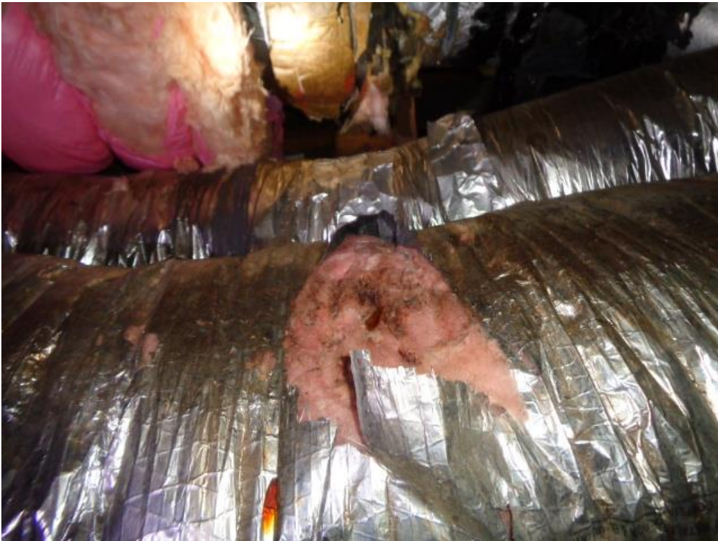
Photo 37: The damaged Mylar ducts in the attic.
