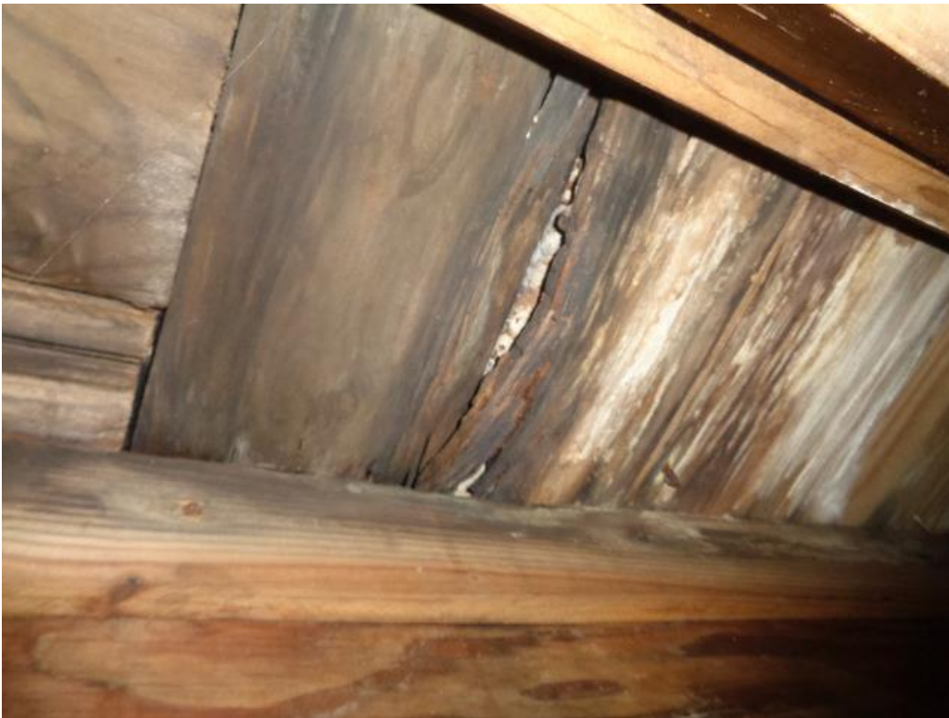
Photo 3: The water damaged subfloor under the front bathroom shower.
