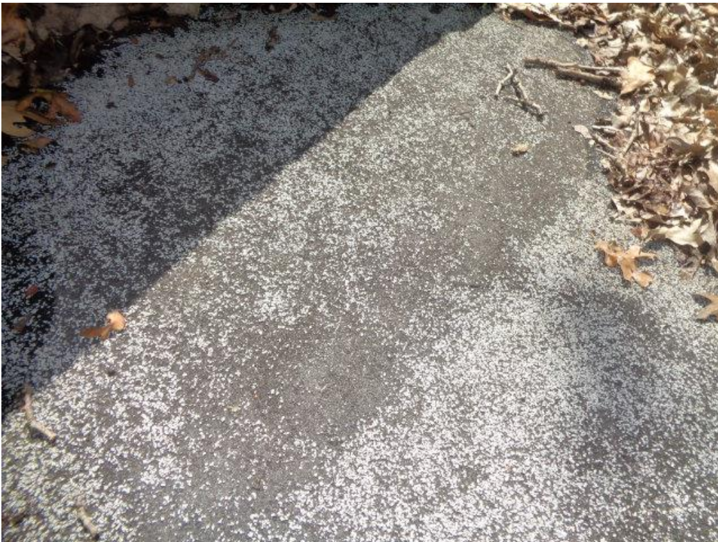
Photo 15: The aged modified bitumen at the flat roof.
