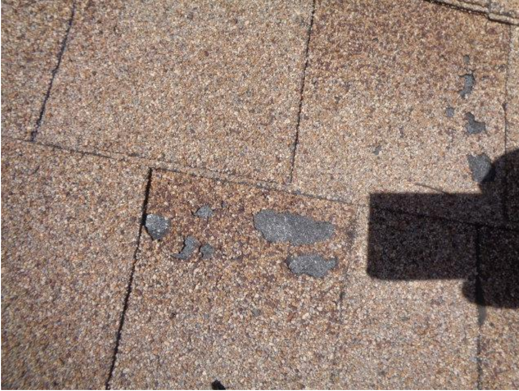
Photo 18: The blistered shingles at the right rear valley area.
