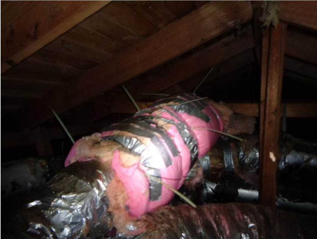
Photo 38: The poorly done repairs to the ducts.
