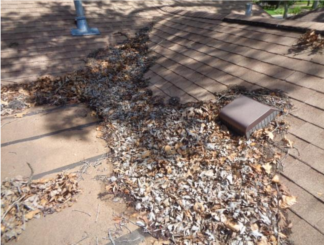
Photo 12: The excessive build up on the roof.
