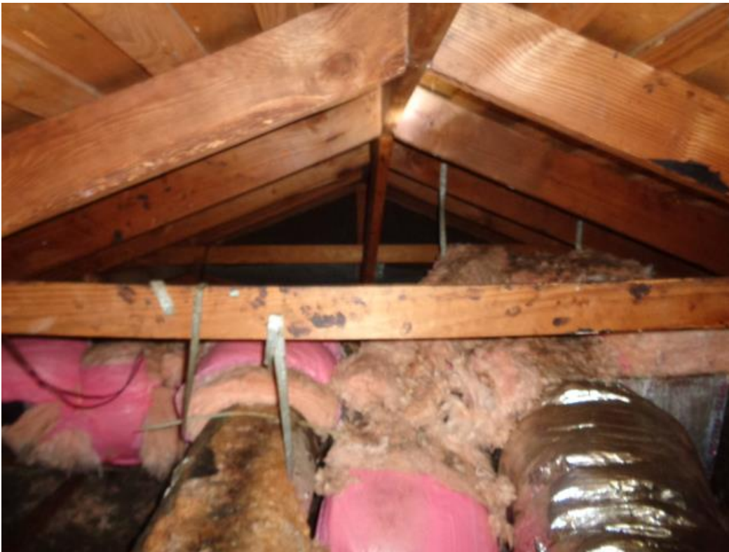
Photo 39: The poorly repaired ducts.
