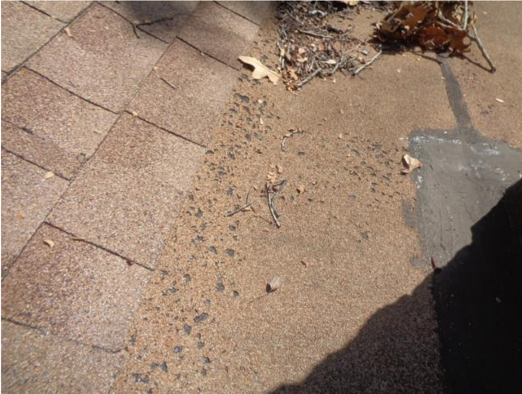
Photo 20: The blistering modified bitumen behind the chimney.
