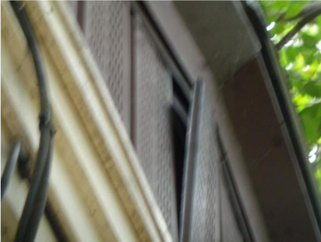
Photo 26: The loose siding at the left rear gable vent.
