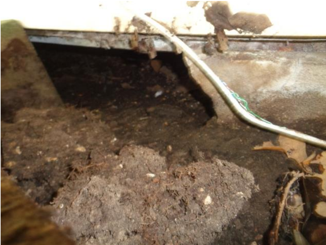
Photo 5: The missing skirting behind the cinder blocks under the rear wall.
