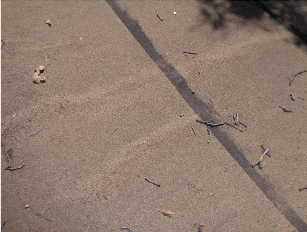
Photo 16: The wrinkling at the modified bitumen at the rear living room low pitched roof.
