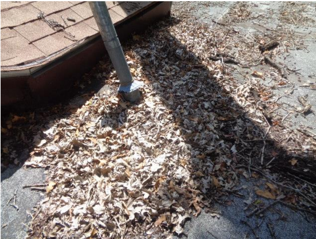
Photo 11: The excessive debris build up on the roof.
