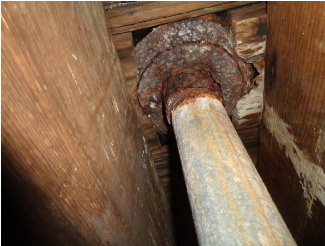
Photo 41: The corroded front bathroom shower drain as seen from the crawl space.
