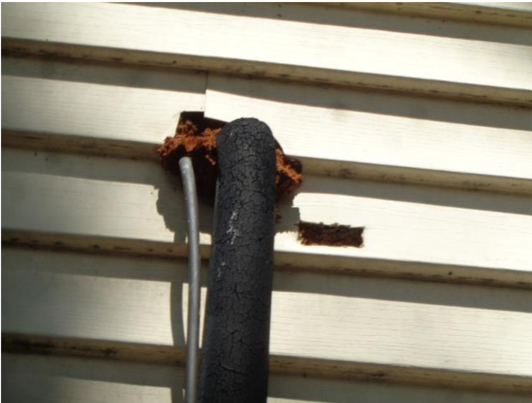
Photo 27: Seal the openings at the left wall siding.
