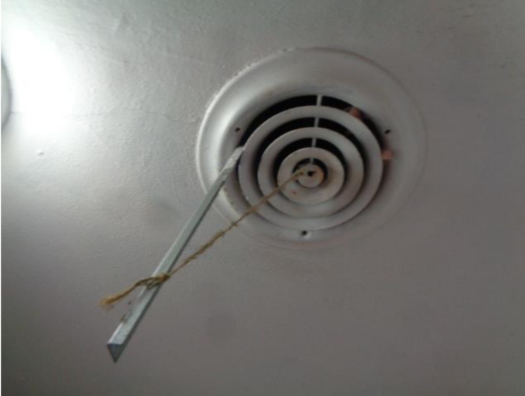
Photo 36: The damper for the kitchen register is held open with a string and a metal rod.
