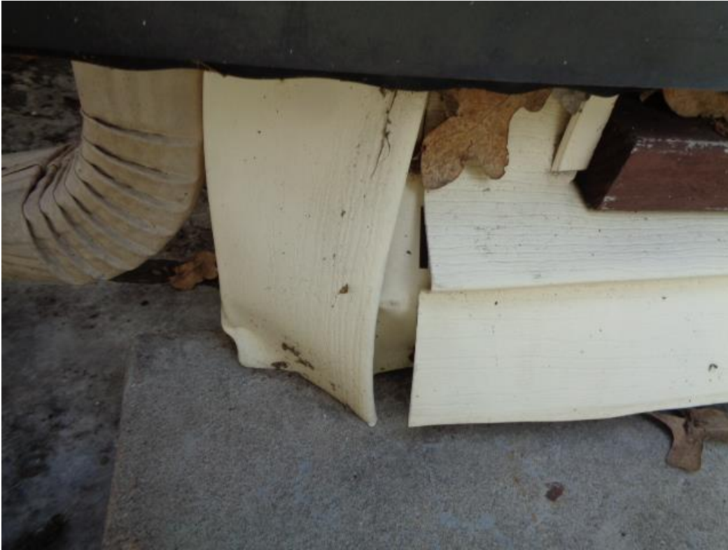
Photo 24: The bent/damaged siding by the rear living room exterior door stoop.
