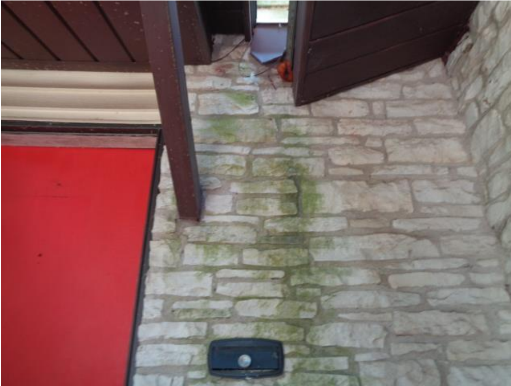
Photo 10: The stains from the roof runoff by the front door.
