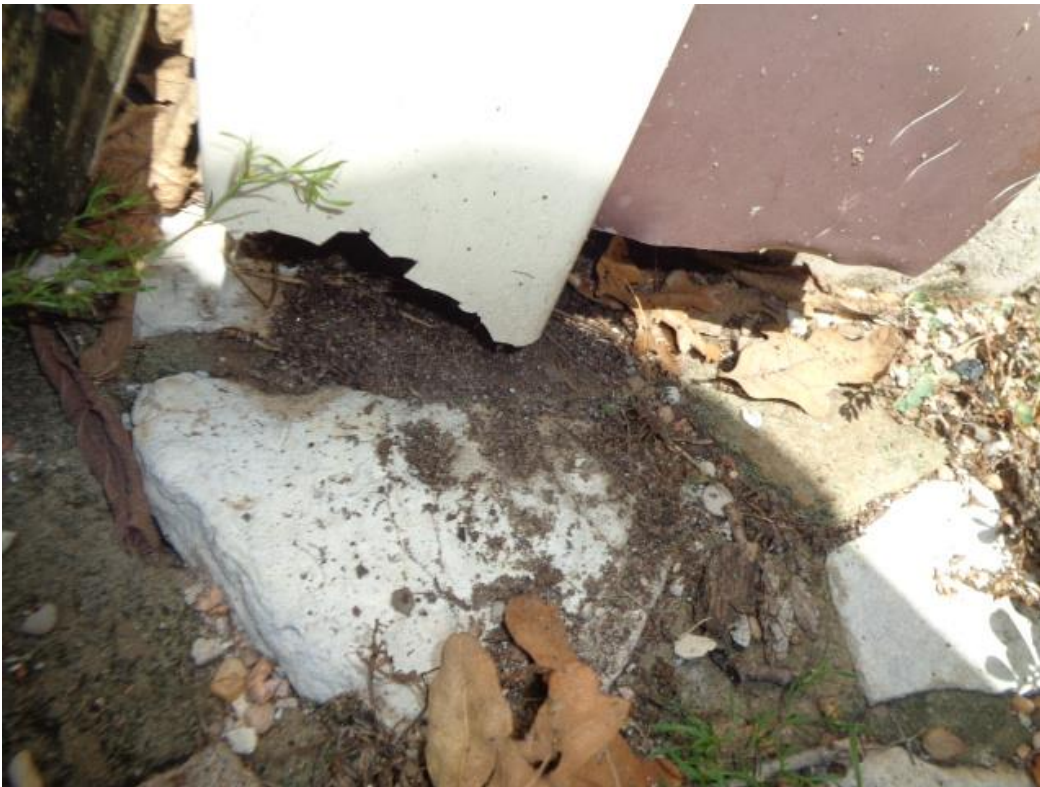
Photo 25: The damaged siding by the storage room exterior door.
