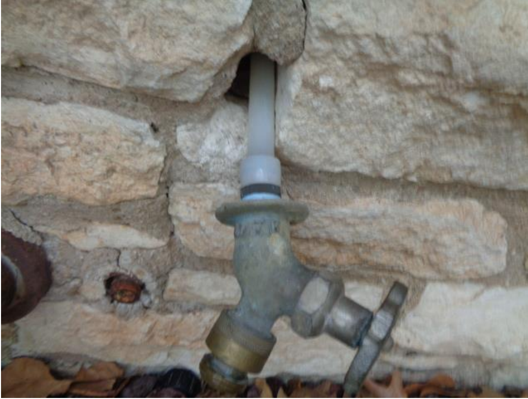
Photo 40: The unsecured, loose, uninsulated water line at the front hose faucet.
