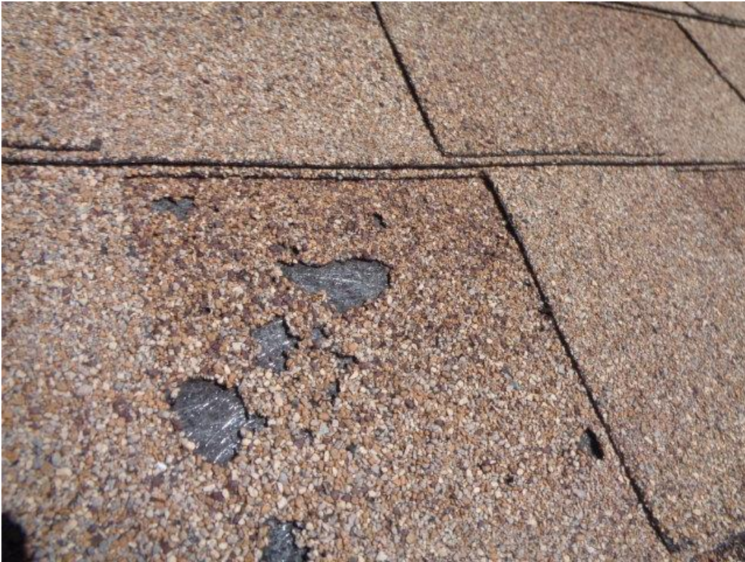
Photo 19: The blistered shingles by the right rear valley.
