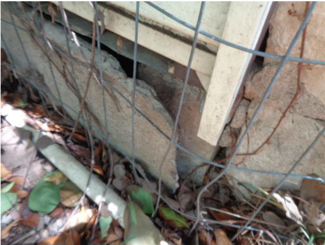
Photo 7: The loose/damaged skirting at the left rear corner.
