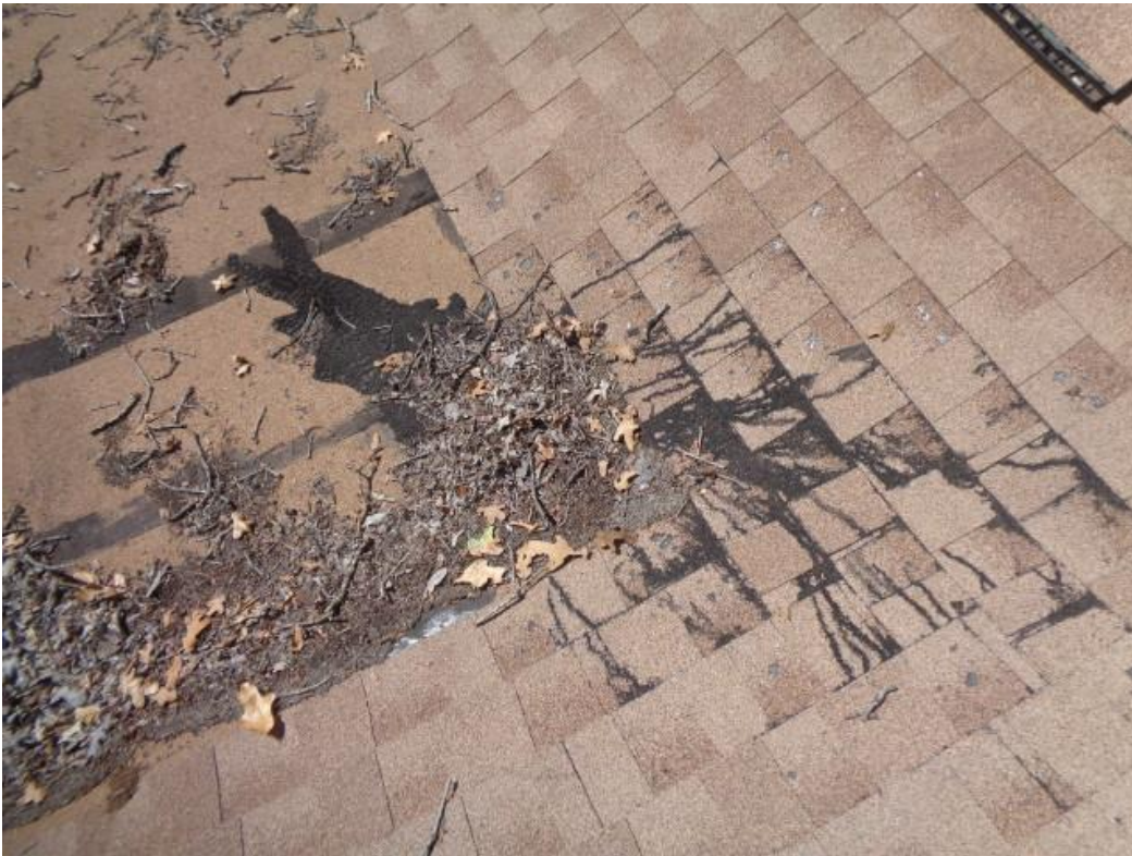
Photo 17: The poorly done repair at the right rear valley.
