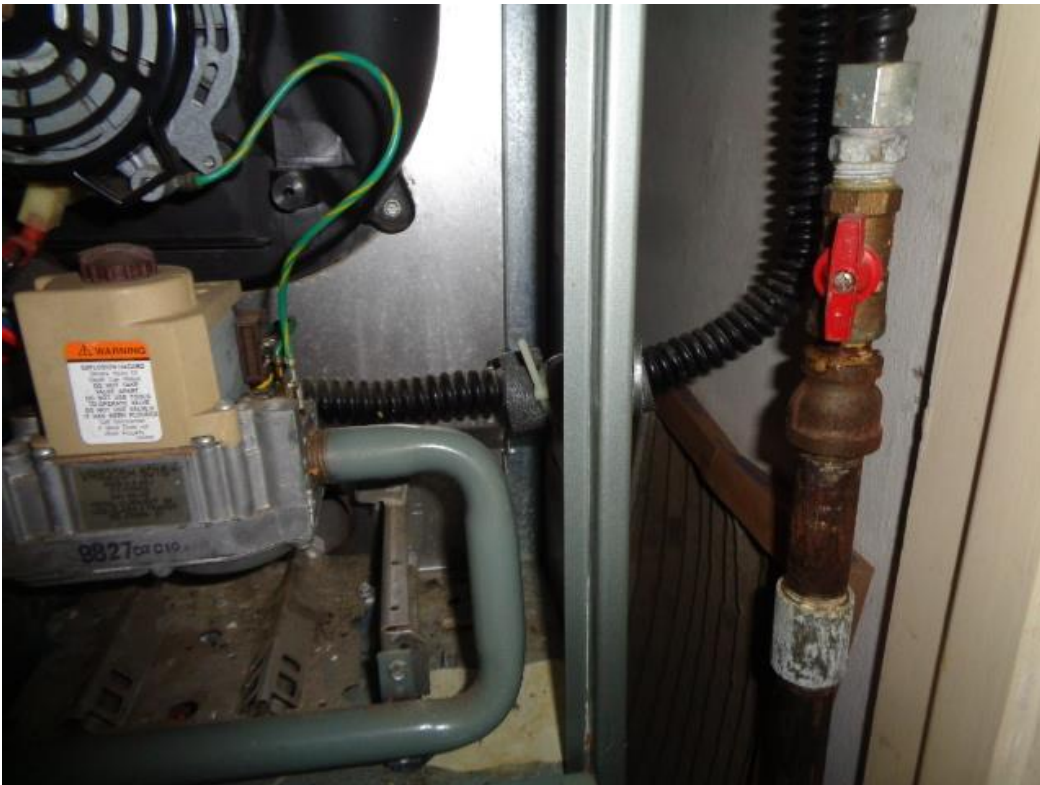
Photo 35: The heater gas line is not rigid pipe as it enters the heater cabinet.
