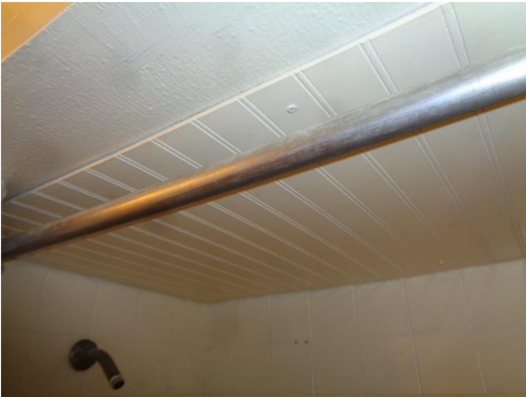
Photo 31: The bead board at the ceiling in the front bathroom shower.
