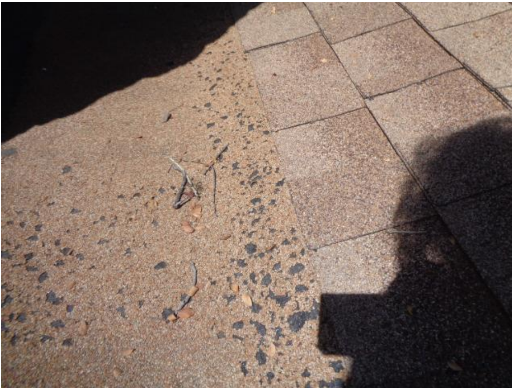
Photo 21: The blistered modified bitumen by the chimney.
