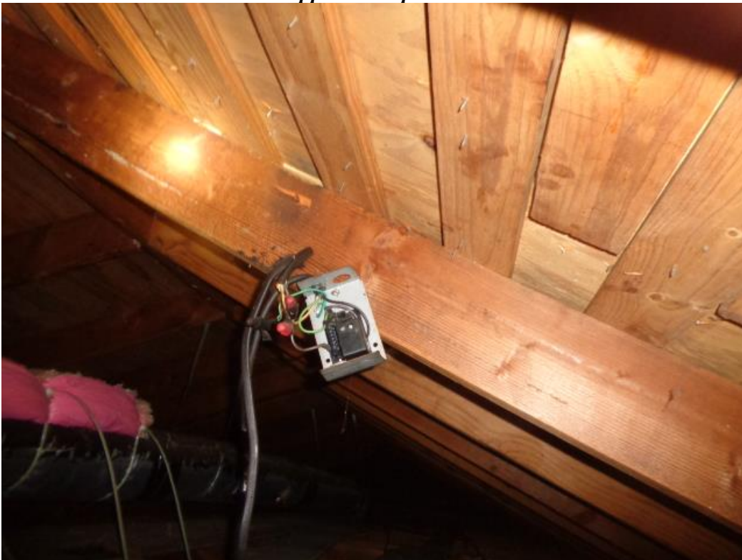
Photo 33: The box that appears to be a fan limit switch with exposed splices in the attic.
