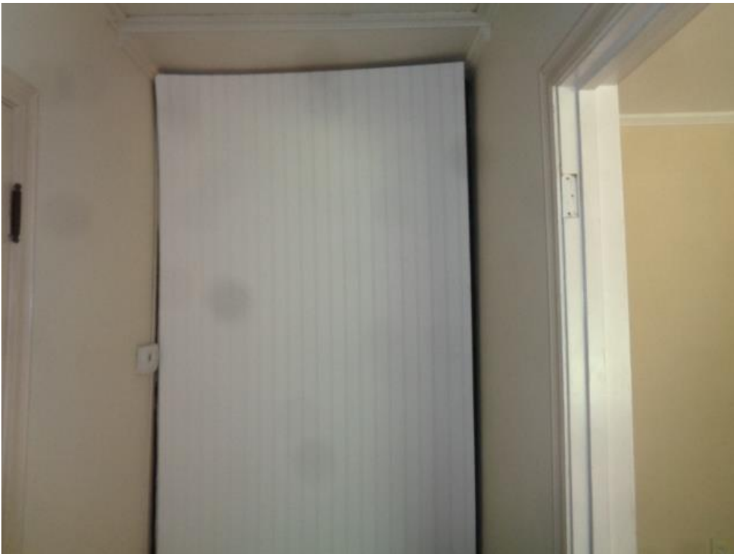
Photo 23: The poorly installed partition in the hall.
