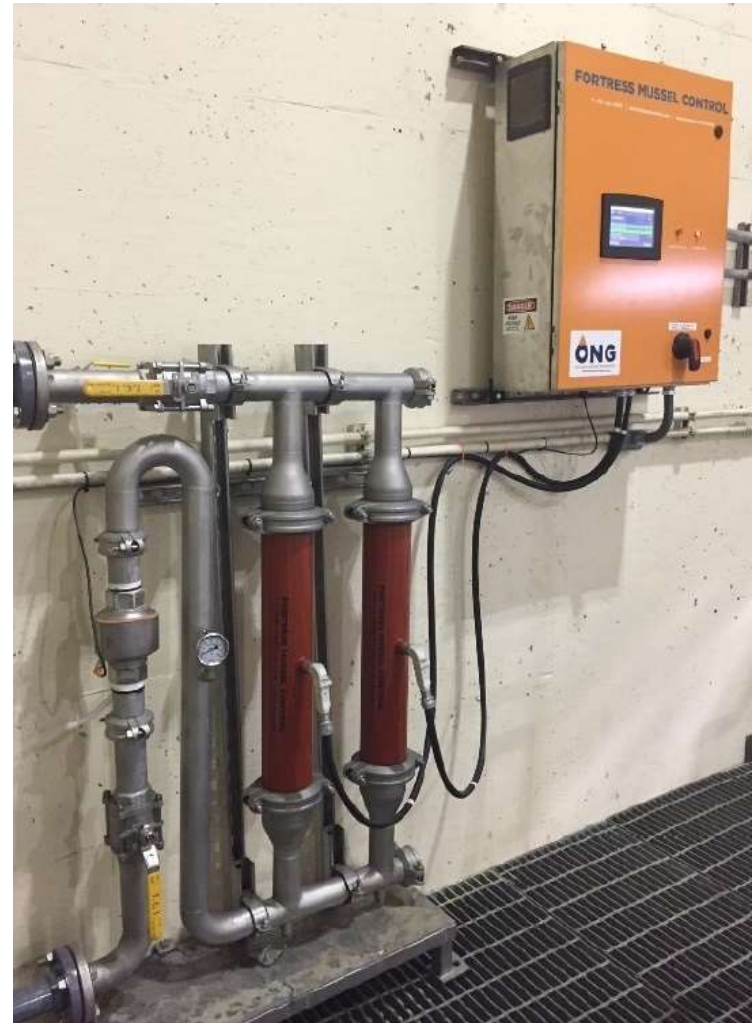
20 MGD Copper Ion Generator Lawrence, KS
