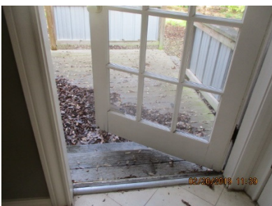
The mud room back door is water damaged.
