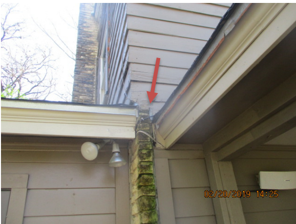
Exposed wall framing on the mudroom back wall is water damaged, partially due to improper installation of the roof flashing above.
