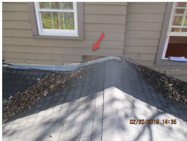
One of damaged areas of the exterior wall siding.
