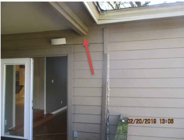
A support post is missing under this patio canopy ceiling beam. Notice the crack in the fascia board above due to partial collapse of the canopy.
