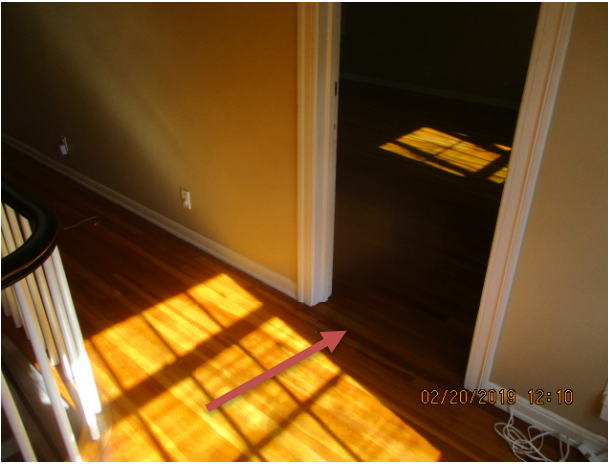
There is a noticeable floor deflection at the entry of the upstairs front right side bedroom due to apparent insufficient floor support.
