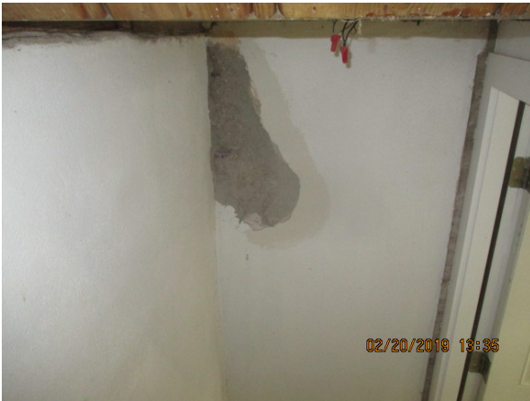
Damaged concrete foundation wall in the garage stairwell
