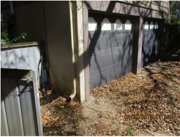
Two photos of the stucco and wood siding on the garage that does not have proper clearance from the soil and concrete surface.
