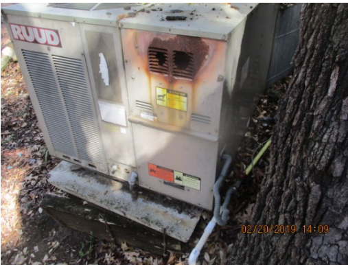
Heat damage to the family room gas furnace.
