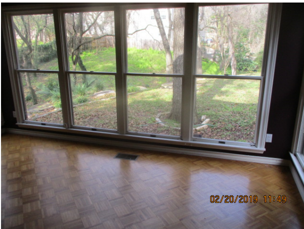
Photo of the window case in the family room back wall. Like the dining room windows, there is considerable water damage to the window case and most window sash.
