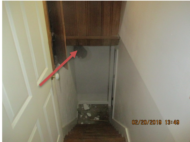
The furdown in the stairwell ceiling is too low.
