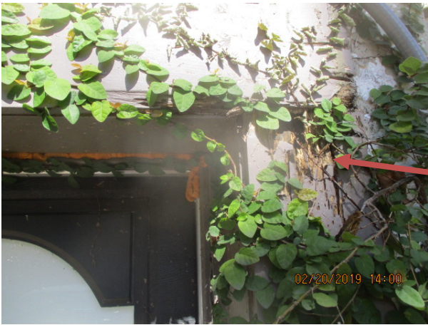
A close up and distant photo of the exposed wall framing at the upper right corner of the garage opening that is water damaged.
