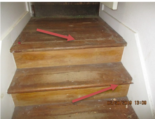
Insect damage to the stairway step treads.
