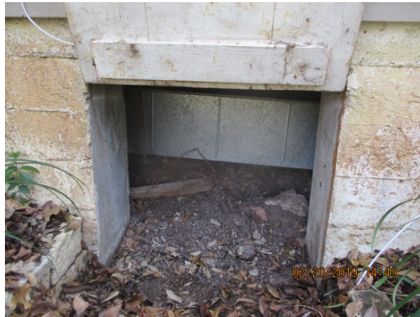
Access to the foundation pier/beam foundation crawl space is blocked by air ducts.
