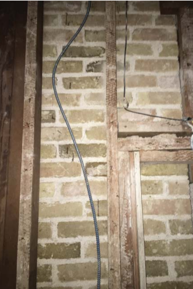
IMAGES OF AUSTIN COMMON MASONRY LEFT EXPOSED AT INTERIOR OF GARAGE AS WELL AS IMAGES OF PAINTED AUSTON COMMON MASONRY AT EXTERIOR OF RESIDENCE.
