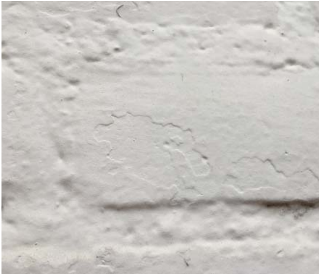
IMAGES OF AUSTIN COMMON MASONRY LEFT EXPOSED AT INTERIOR OF GARAGE AS WELL AS IMAGES OF PAINTED AUSTON COMMON MASONRY AT EXTERIOR OF RESIDENCE.
