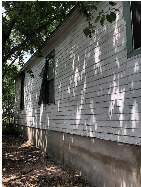
6. Significant portions of remaining Original siding are beyond repair due to dryrot/deterioration/damage; portions have been replaced with newer materials 7. Additional windows not consistent with original construction
