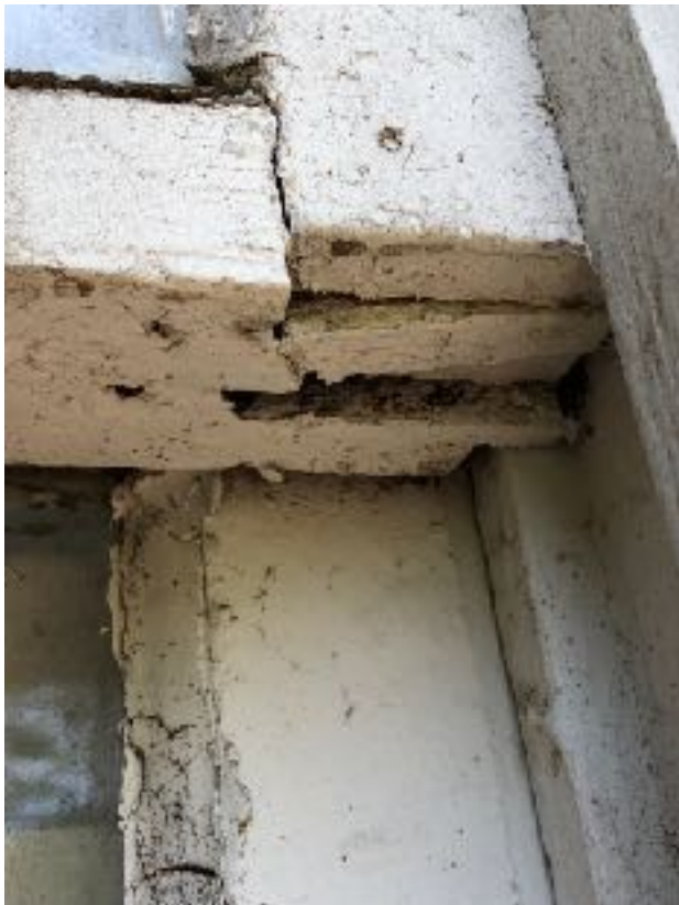
Image of window condition 1410 West 9th Street (this page). Evidence of Rot, Termite damage, and physical damage present.
