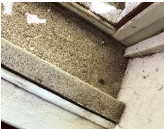
Image of window condition 1408 West 9th Street (this page). Evidence of Rot, Termite damage, and physical damage present. Damage to existing windows due to plexiglass reinforcement and lack of weatherstripping causing further moisture damage at window frame.
