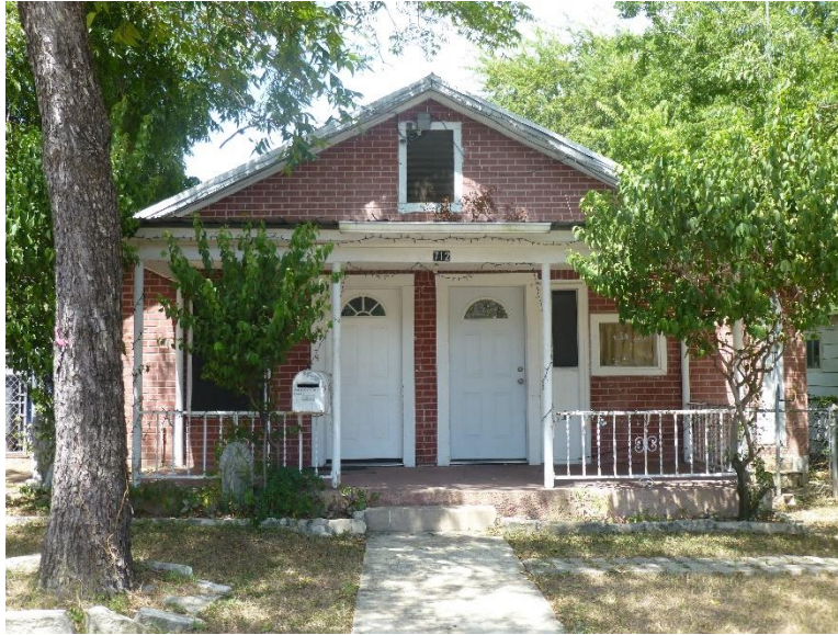
Primary (south) façade elevation of 712 W. Monroe Street.
