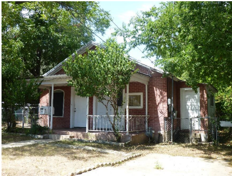
Primary (south) façade and east elevation.
