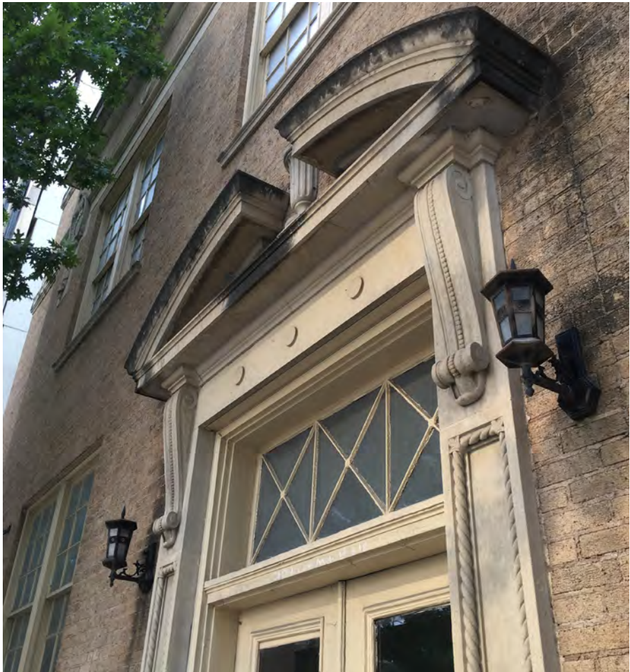
LIMESTONE DETAILING AT EAST ENTRY
