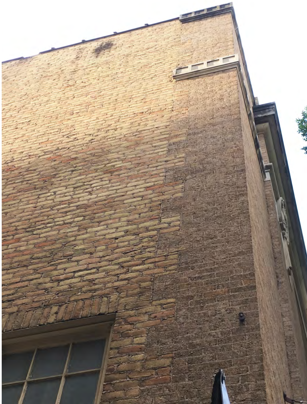
SOUTHEAST CORNER, SHOWING TWO TYPES OF BRICK
