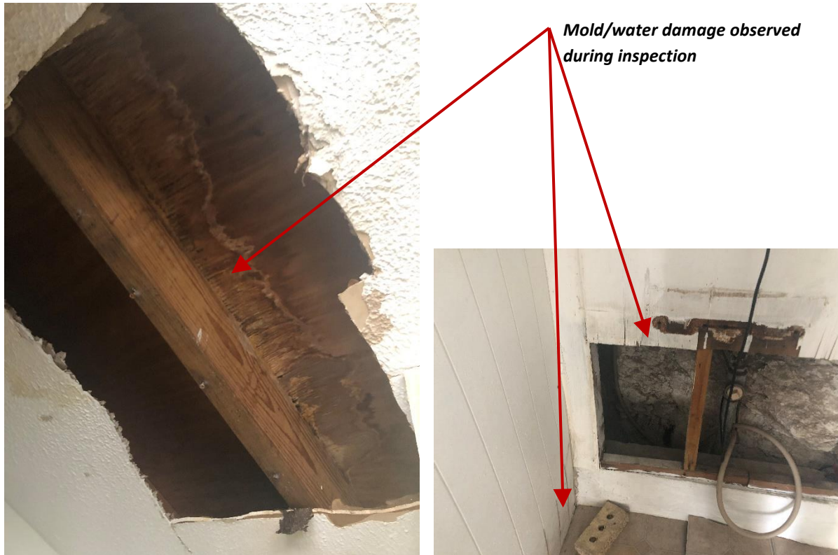
Figure 6. Mold and framing deterioration
