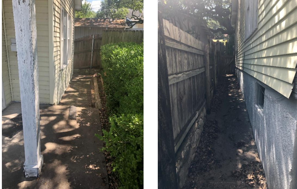
Figure 2. Site Drainage. Inadequate drainage and walls limiting water runoff
