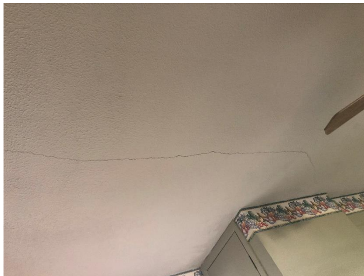
Figure 5. Multiple cracks in ceiling.
