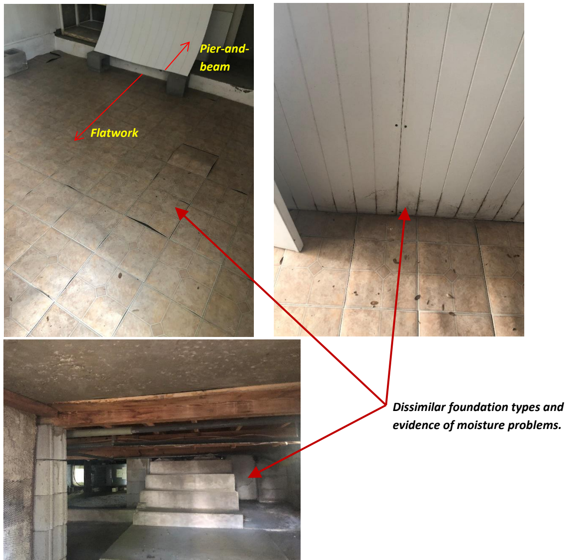
Figure 3. Dissimilar foundation types
