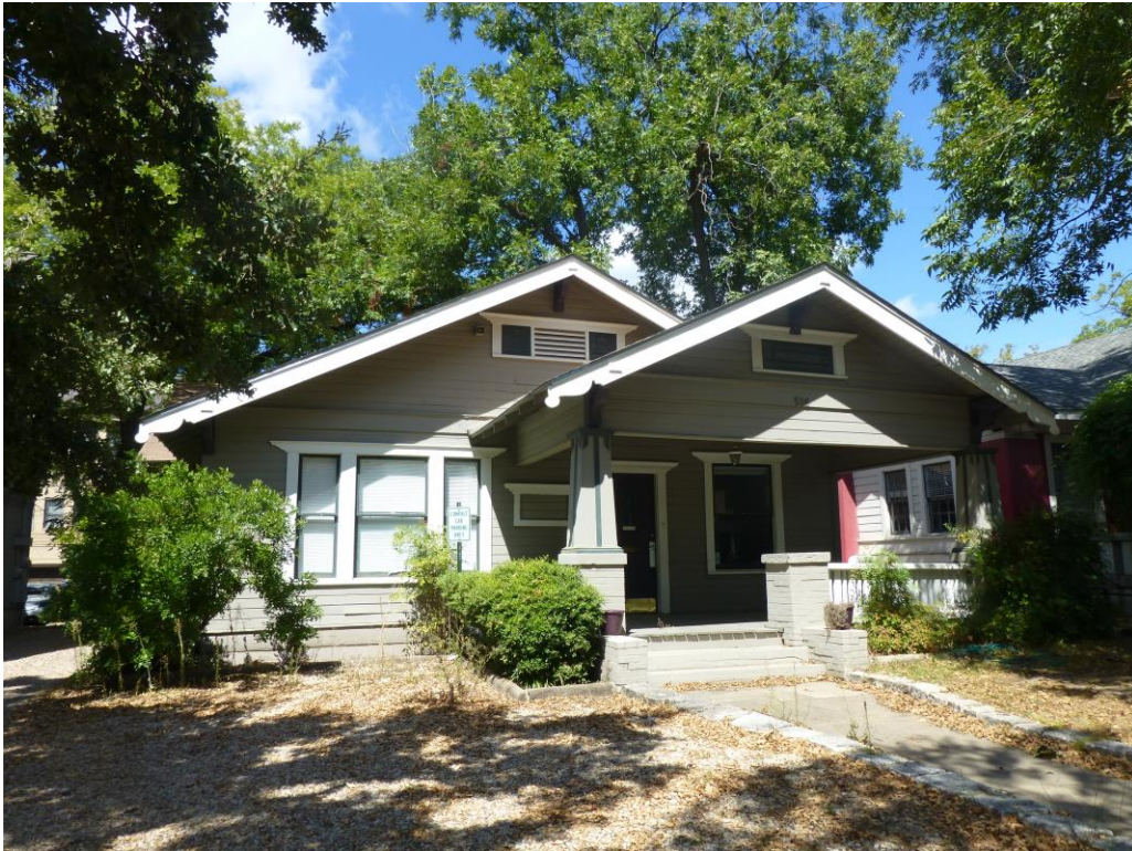
Primary (east) façade of 506 Oakland Avenue.
