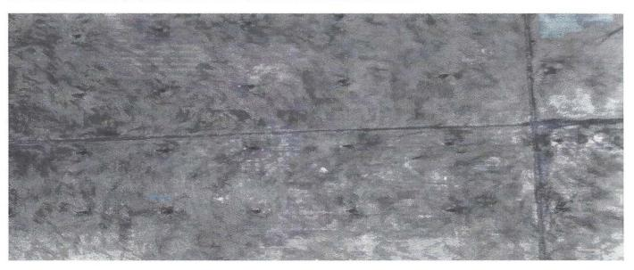
The picture above is close view of the Filter Plate located under the drain and the area that will need to be hydro-blasted. These Filter Plates are 22' wide by 36' long, and the holes are 0.125" in diameter (as reference in Section 0500 paragraph 5.3 and 5.4).
