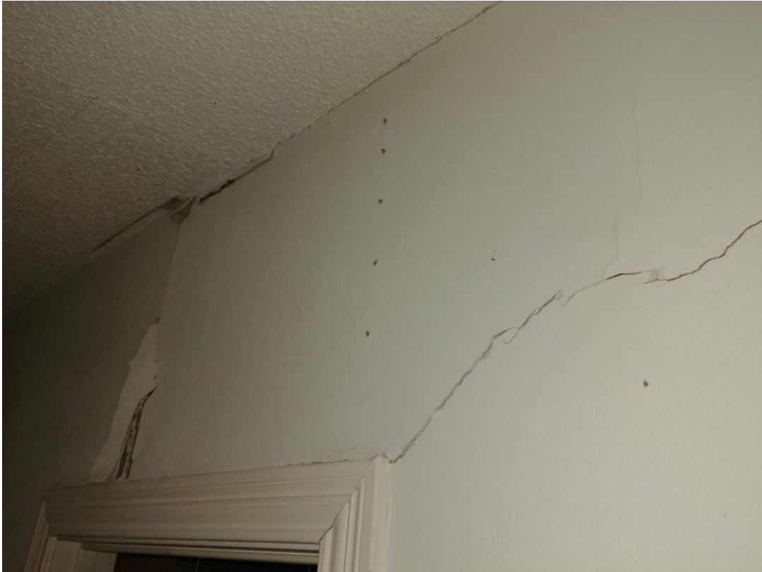
Interior cracks
