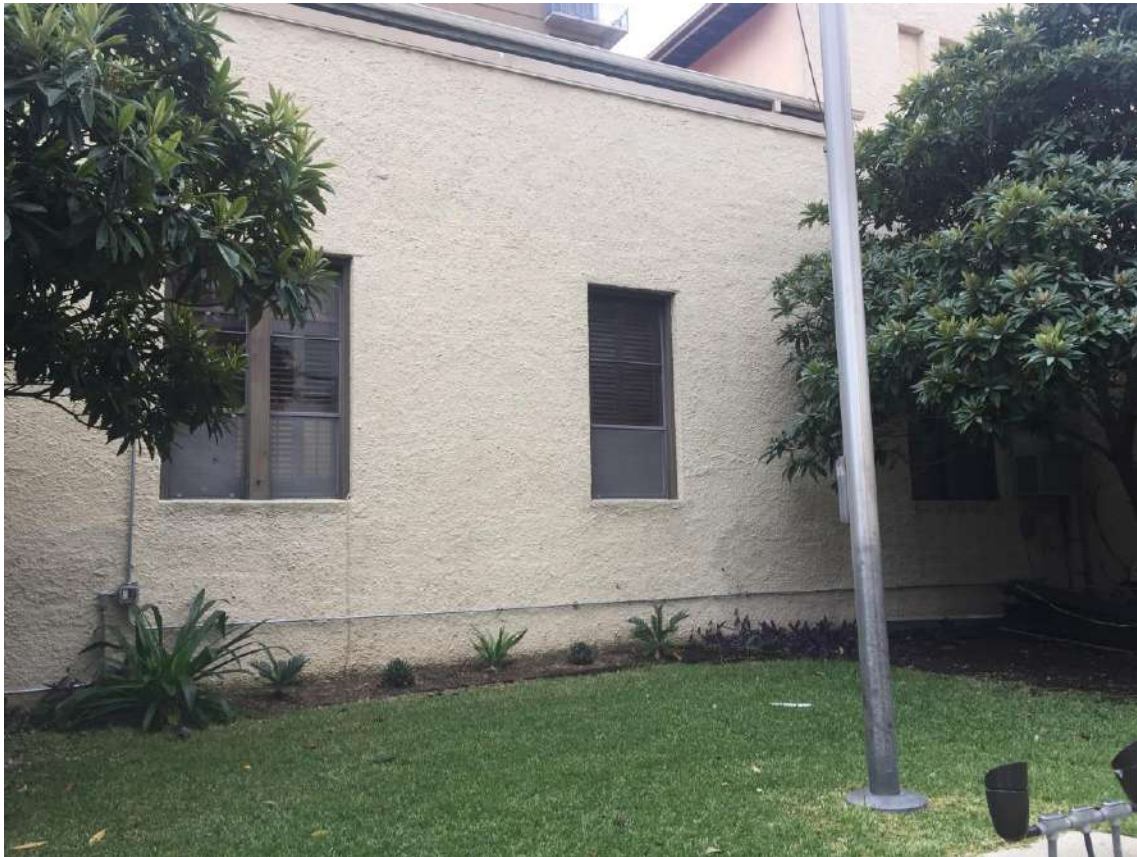
Aluminum windows and rotted frames replaced with era-appropriate windows
