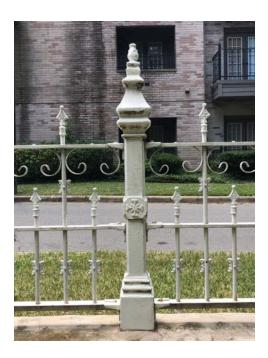
New molds will be produced to replicate the original cast iron posts. Posts are 42 in. tall. The cross motif was appropriate to the fence's original funerary setting in a 18<sup>th</sup> century Seguin cemetery.
