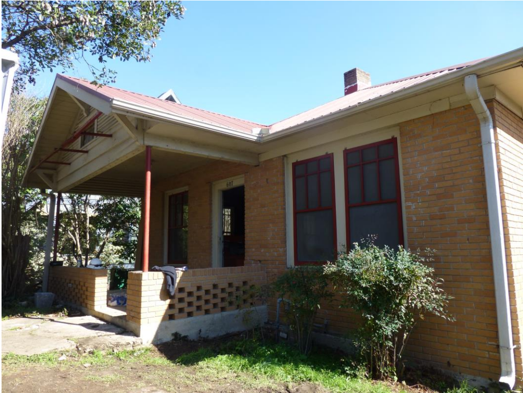
Primary (west) façade of 607 Oakland Avenue.
