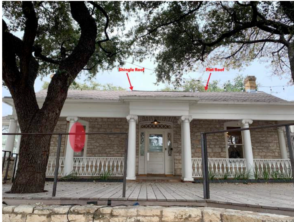
Shingle roof and flat roof identified above. Windows to be replaced marked in red.
