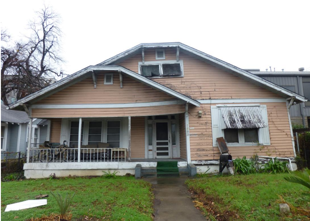
Primary (north) façade of 1603 E. 7 th Street.
