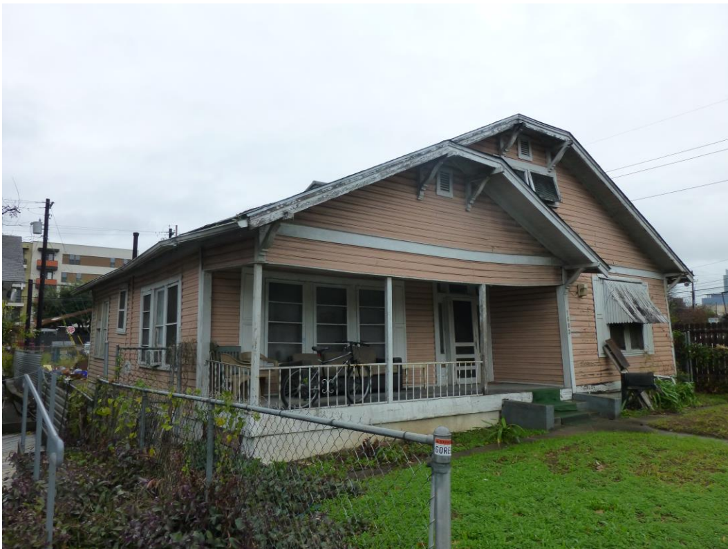
East elevation and north façade.
