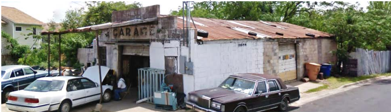
Google Street View image from 2009 shows missing canopy
