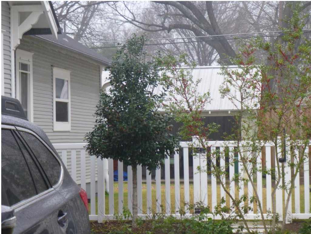
Detached garage at 4010 Avenue G.
