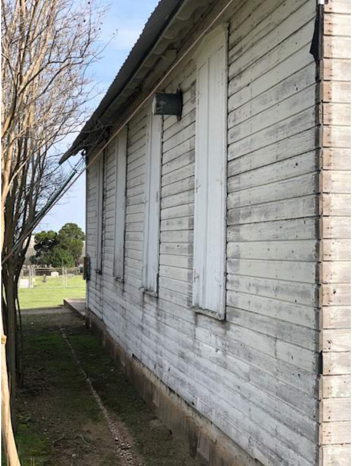
North side view shows steel bracing, stove chimney flue.
