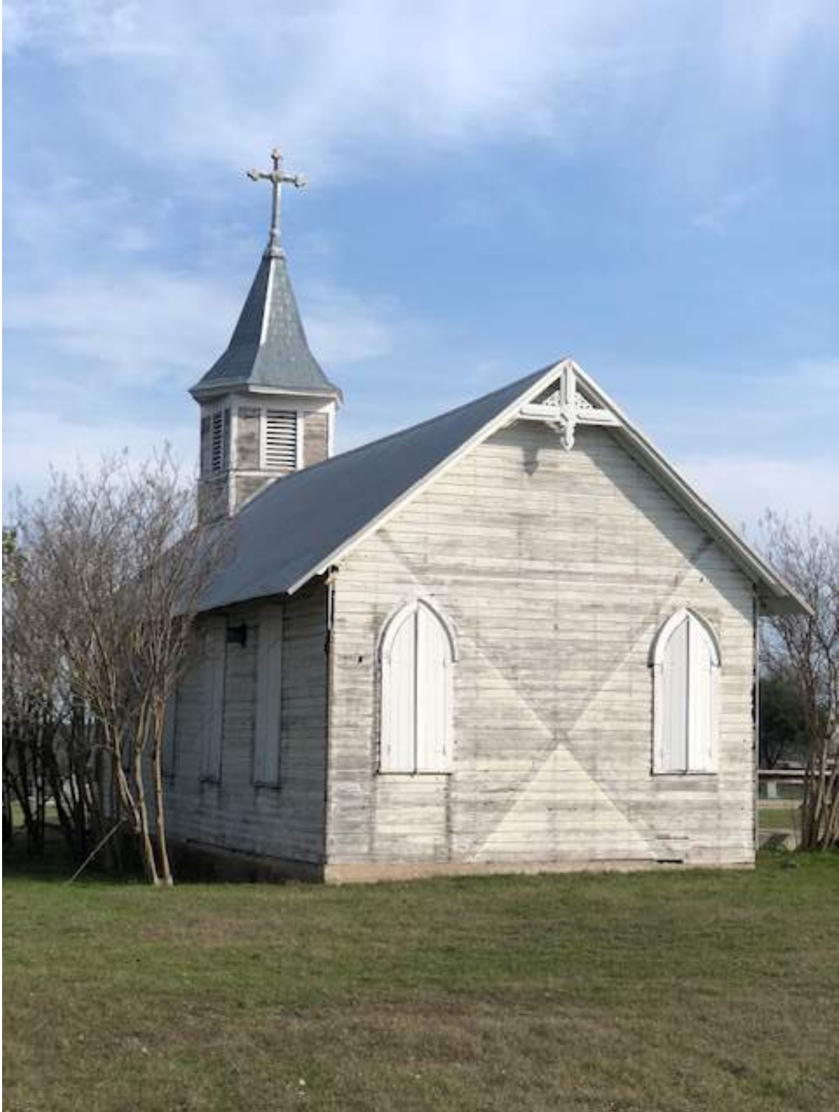
Rear elevation shows shadow from onetime braces, original location of back door.
