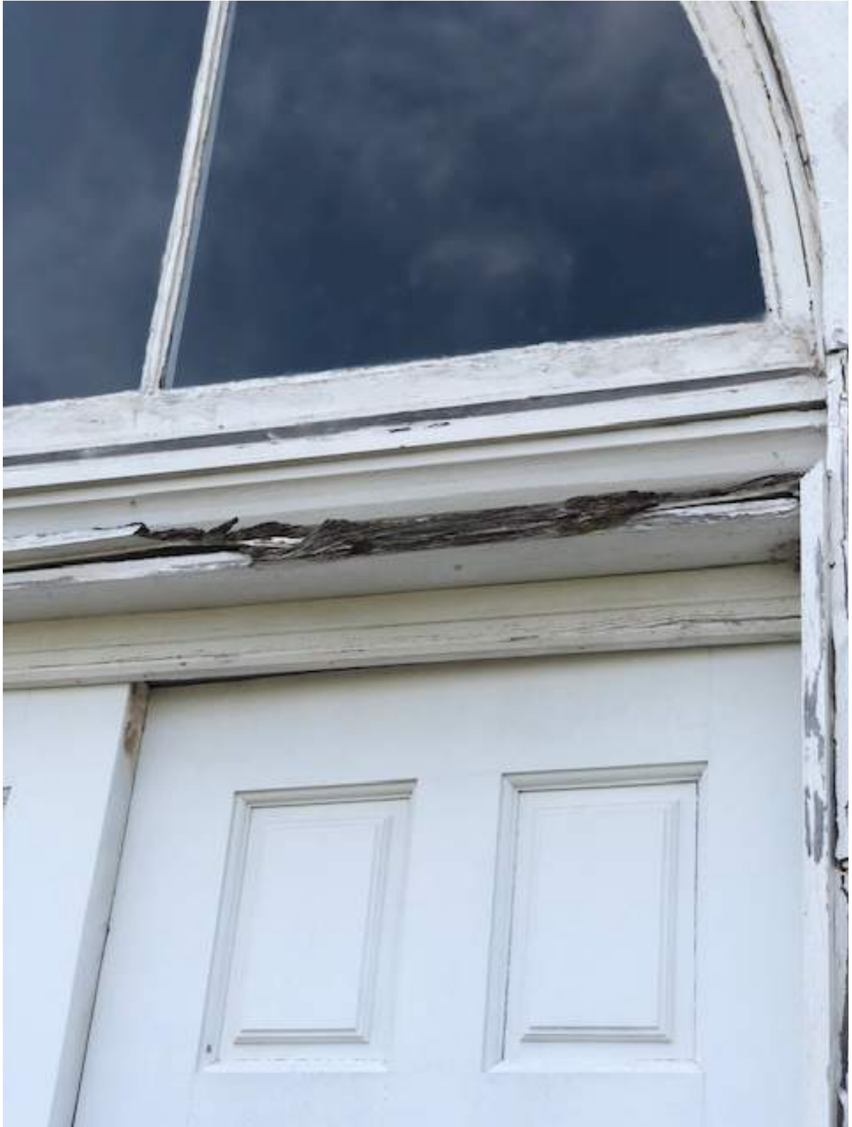
Trim detail at the front double door.
