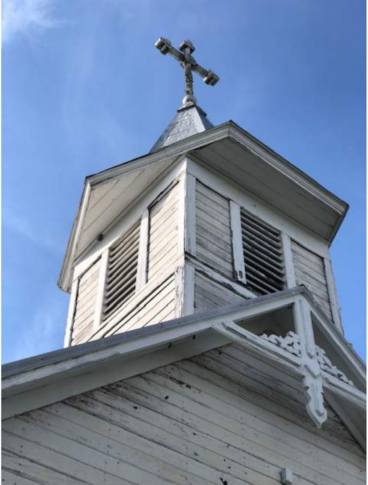
Belfry detail shows louvers, fretwork and cross.
