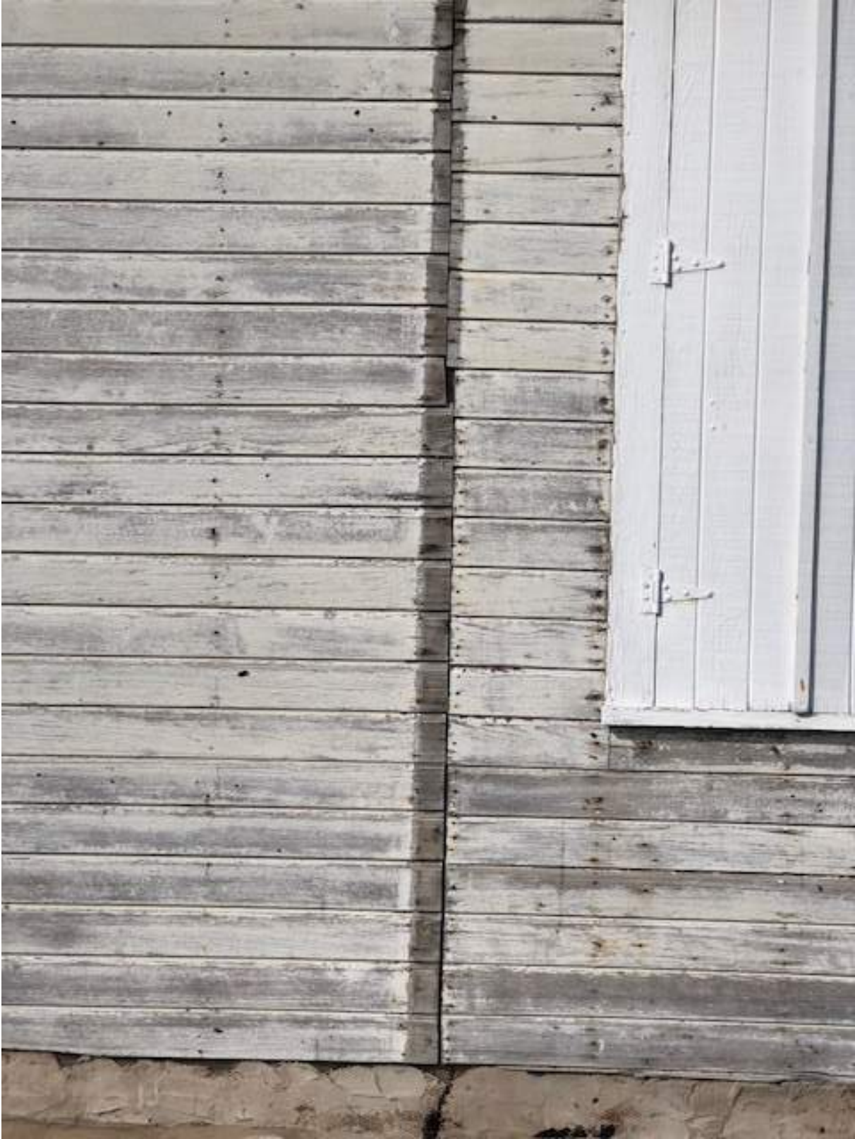
Siding joint shows where front was added on in 1890s
