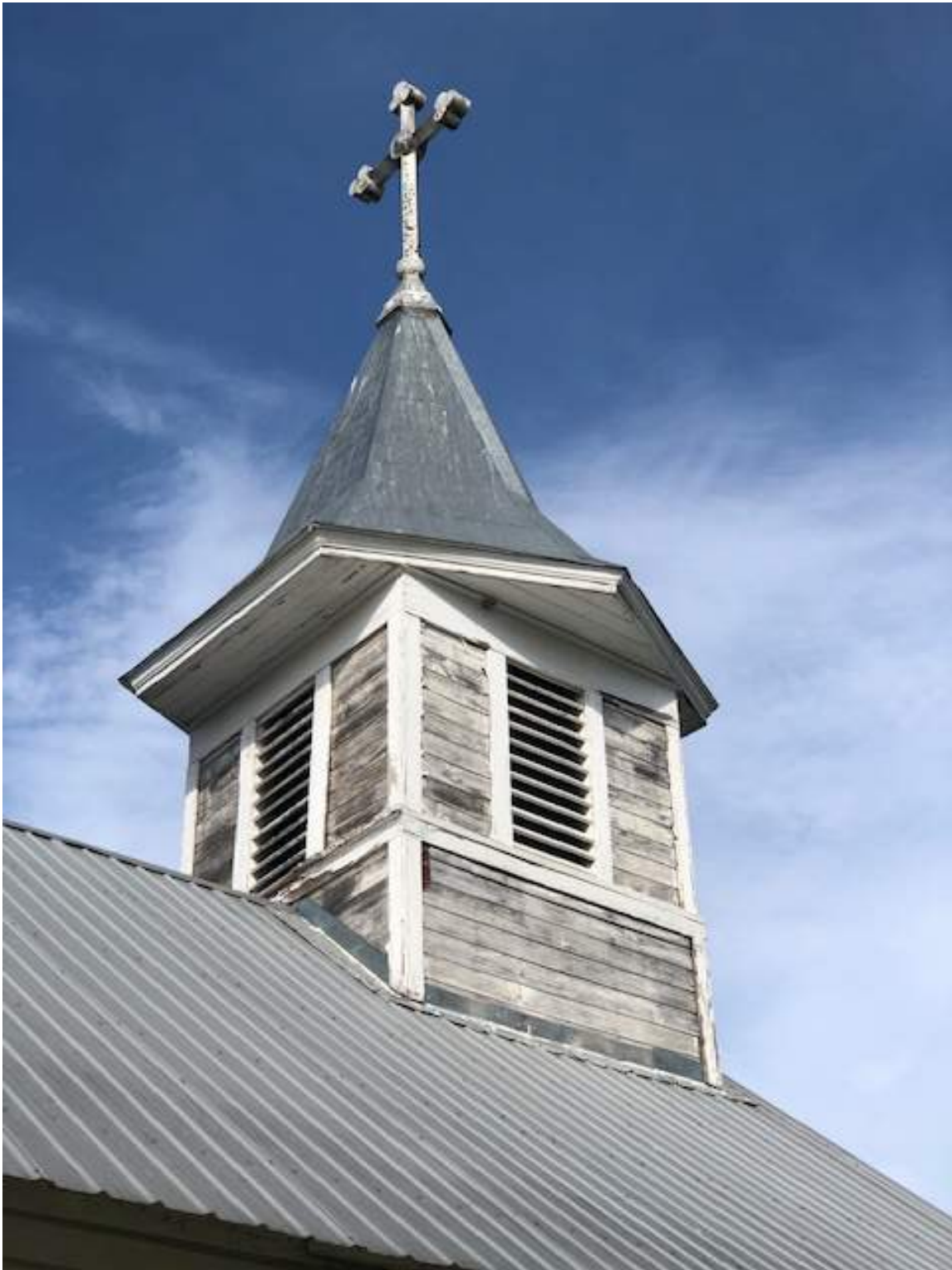
Belfry detail shows current condition.
