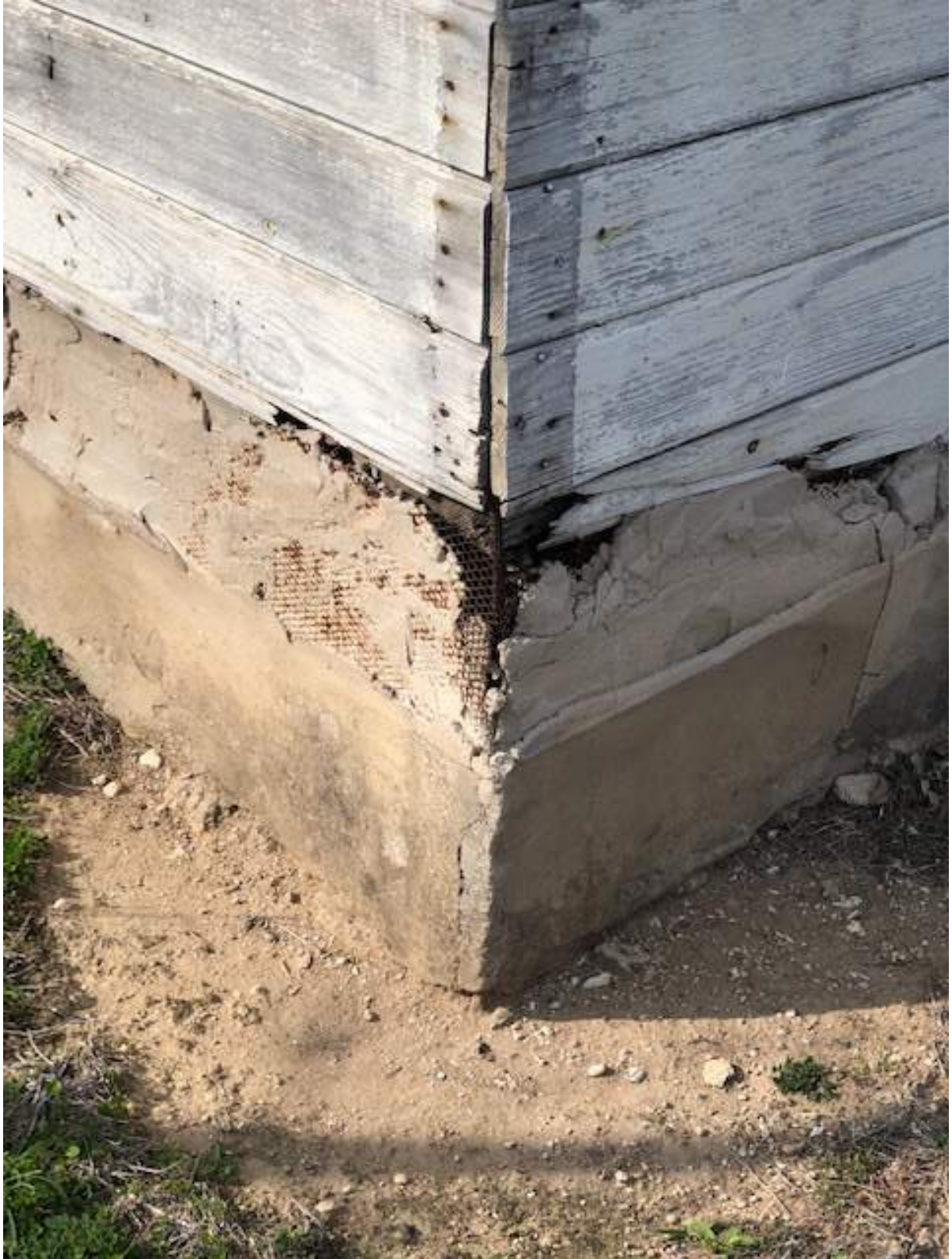
Foundation detail at the front right corner.
